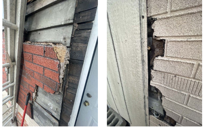
Site Photos 8-9, by Applicant: (Southwest) rear elevation showing wood clapboard beneath insul-brick and application of wood paneling
