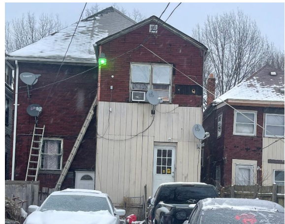
Site Photo 5, by Applicant Jan 2022: (Southwest) rear elevation showing previous insul-brick siding and new wood panel siding.
