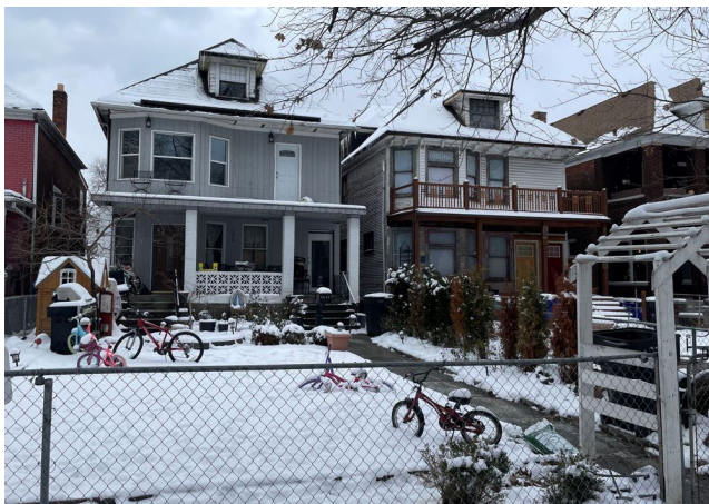
Site Photo 1, by Staff January 25, 2022: (Northeast) front elevation, showing arbor, removed tree, and new installed siding.
