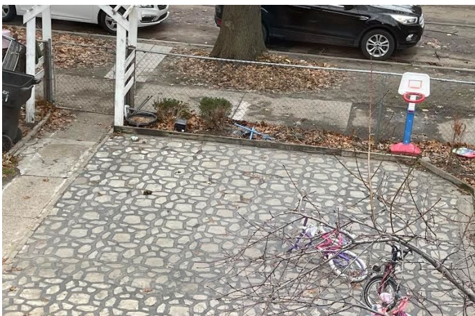
Site Photo 4, by Applicant: (Northeast) front yard showing installation of pavers, raised garden beds, and arbor.
