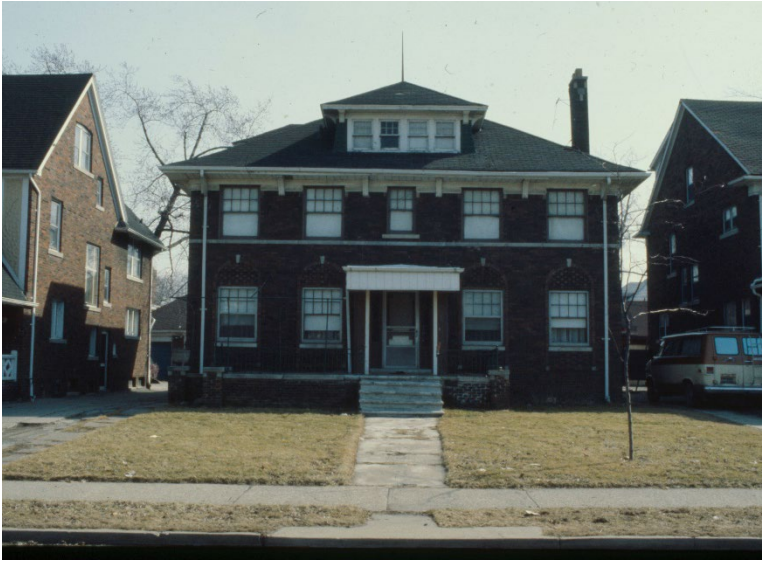
Historic photo, by HDAB 1980: (Northwest) front elevation.
