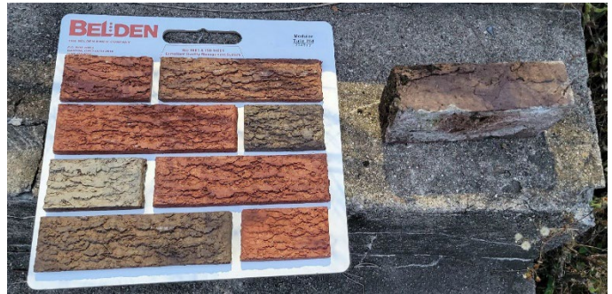
Sample photo, by Applicant showing existing brick (right) and sample brick proposed for in-fill of rear door.
