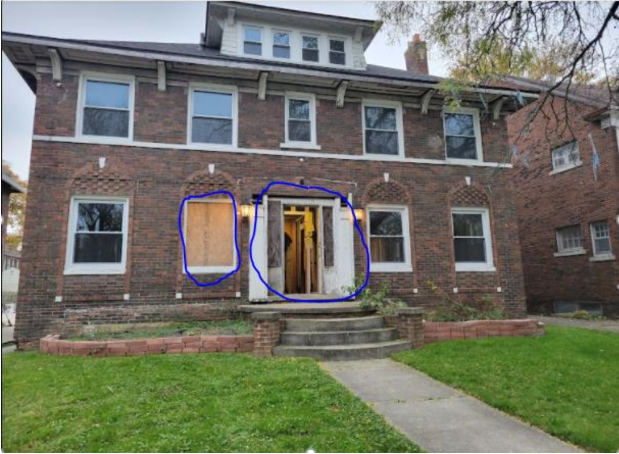
Current State of Home, Windows and roof replaced
