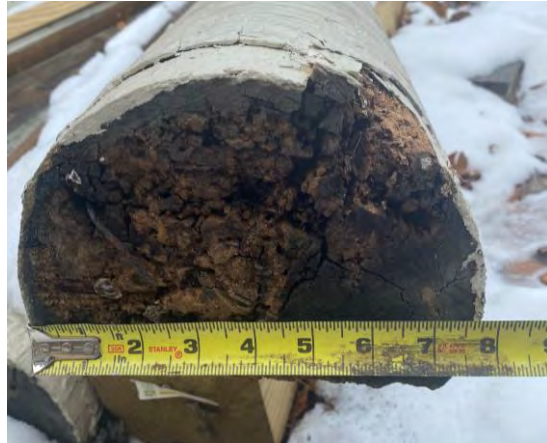
Bottom diameter of pilaster – eight inches
