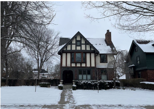
Site Photo 1, by Staff January 25, 2022: (Southwest) front elevation.
