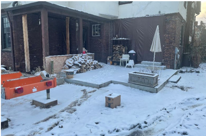
Site Photo 3, by applicant: (Northeast) rear elevation showing location of proposed addition.
