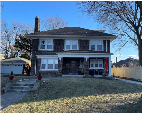
Site Photo 1, by Staff January 21, 2022: (North) front side
