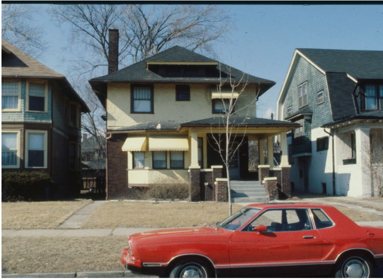
Site Photo 3, by HDAB 1980: (Southeast) front elevation
