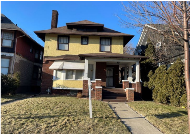
Site Photo 1, by Staff January 21, 2022: (Southeast) front elevation.
