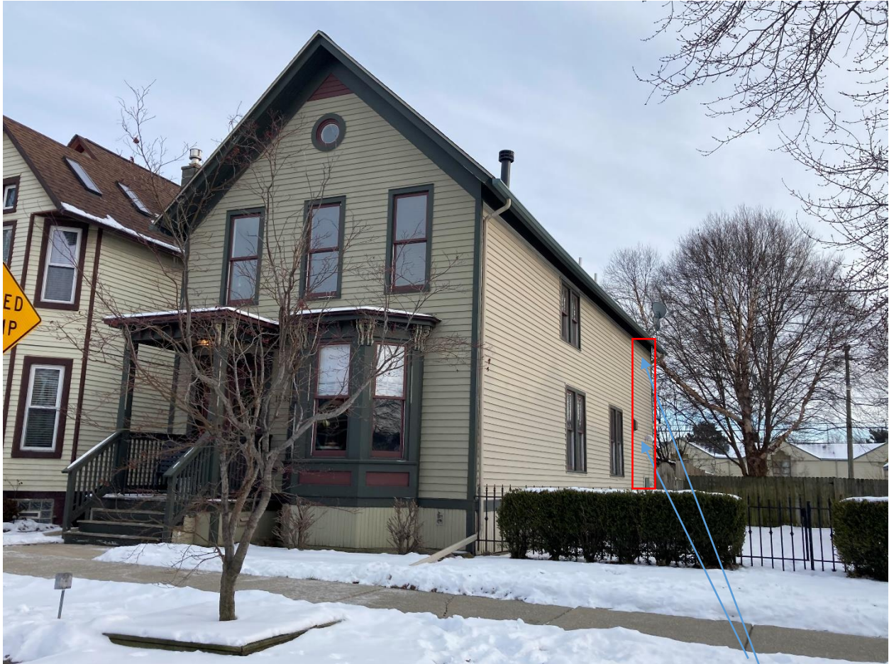
1535 Leverette, current appearance, New vinyl-clad windows to be installed at these locations. Area outlined in red shows location of 1985 addition
