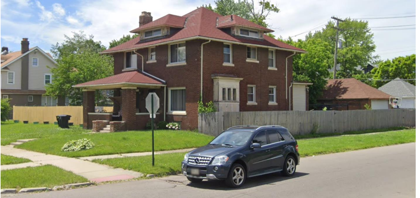
1404 Atkinson, 2019 Google Streetview image, appearance prior to fire
