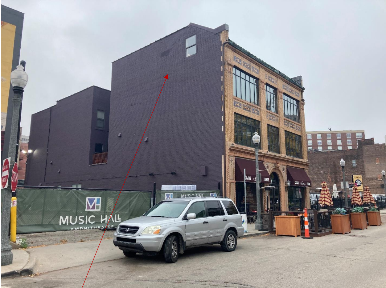
1502 Randolph, staff photo taken 10/7/2021, view of the north/side elevation. The new digital billboard will be installed at this location, beneath the window at the north elevation
