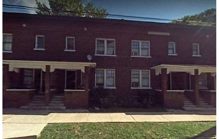
Site Photo 4, by Google Street August 2007: (Southwest) front elevation showing previous windows, and paint-free capstones and sills.
