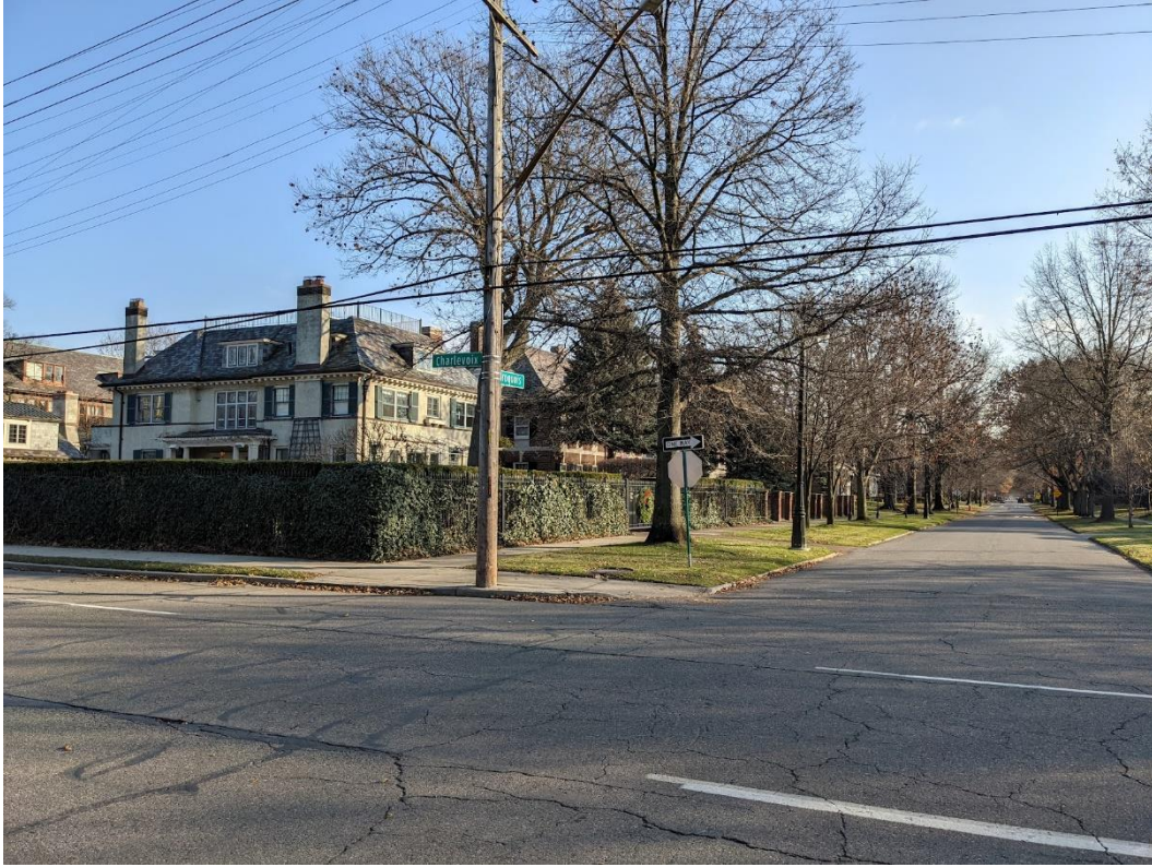
Southeast corner of Iroquois and Charlevoix, Condition "A", full transparent fence (grown in)
