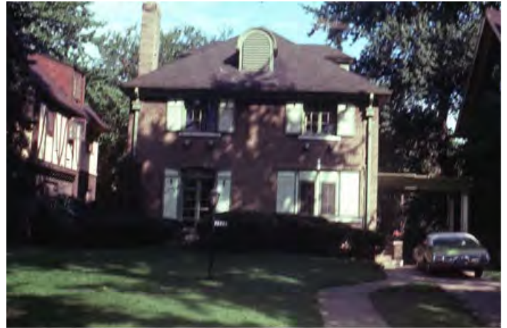
Site Photo6, designation slide 1974: (South) front elevation showing front elevation shutters and wood paneling.
