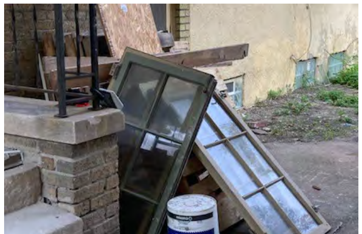
Site Photo 5, by Staff August 5, 2021: (Southeast) front/side showing original wood casement windows.
