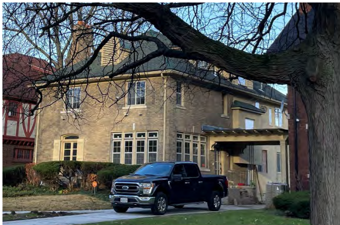
Site Photo 4, by Staff November 18, 2021: (Southeast) front/side elevation showing windows replaced.
