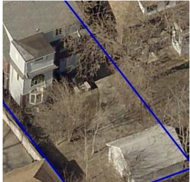
2018 Pictometry photo Two-car garage still intact.
