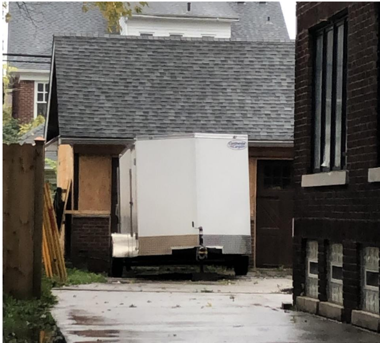
View from Longfellow. HDC staff photo, October 29, 2021
