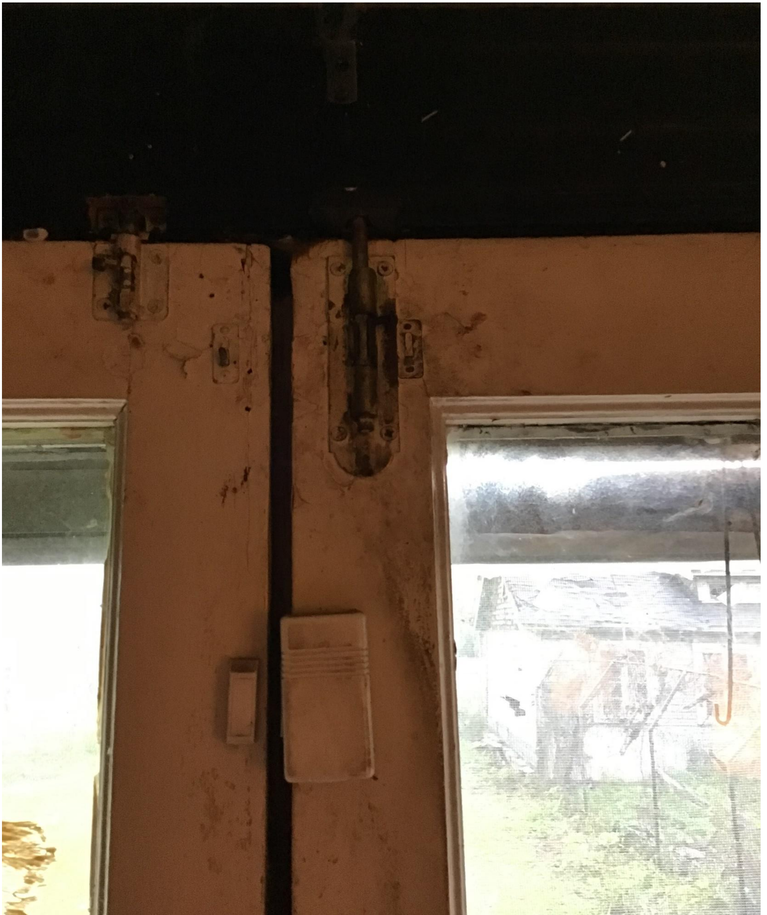
Several barrel bolts are used to keep door lock/shut
