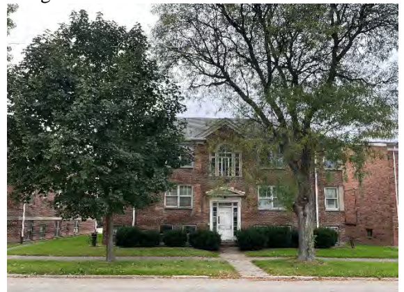
Site Photo 2, by Staff October 22, 2021: (East) front elevation of 9710 W Outer Dr.
