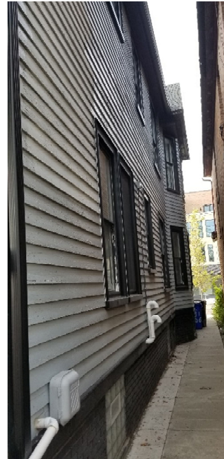
East Elevation (view towards North)
