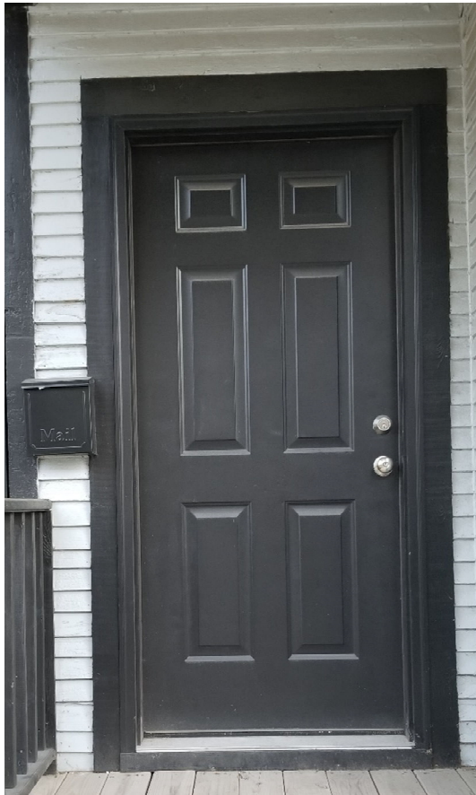
Existing Front Door
