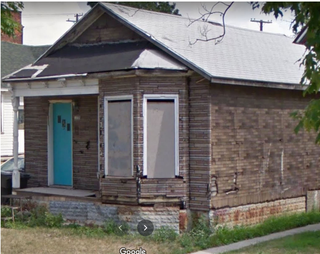
Google Street View shows property with incompatible asphalt siding as it appeared in July 2016.
