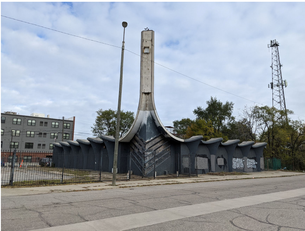
View of existing conditions at 2238 Wabash. Staff photo, November 2, 2021.
