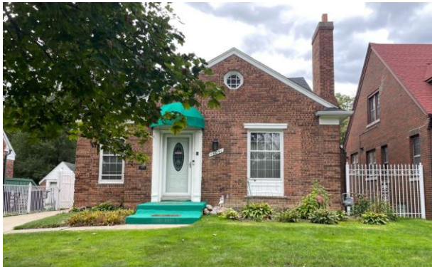
Site Photo 1, by Staff October 22, 2021: (East) front side
