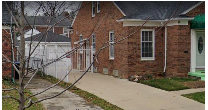
Site Photo 2 by Google Street Nov.2020: Demolished Garage (Southeast).
