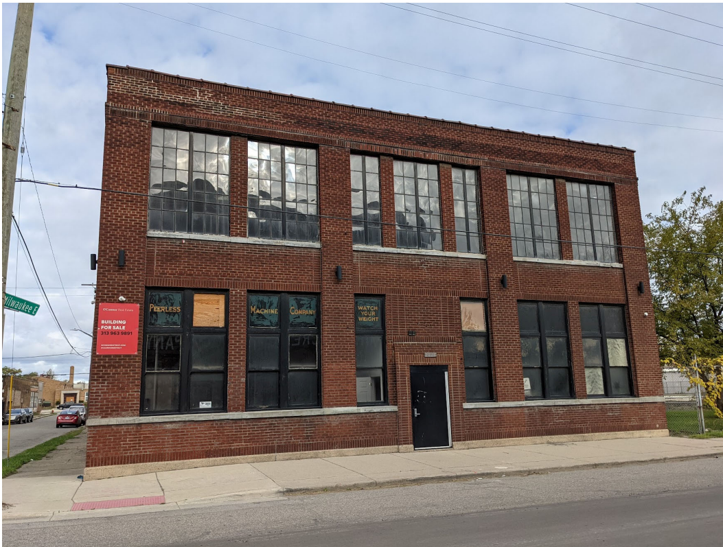
View of primary (front) elevation. Compare to proposal rendering, next page. Note juxtaposition of triple-sash wood windows with steel shop windows above. Staff photo, November 2, 2021
