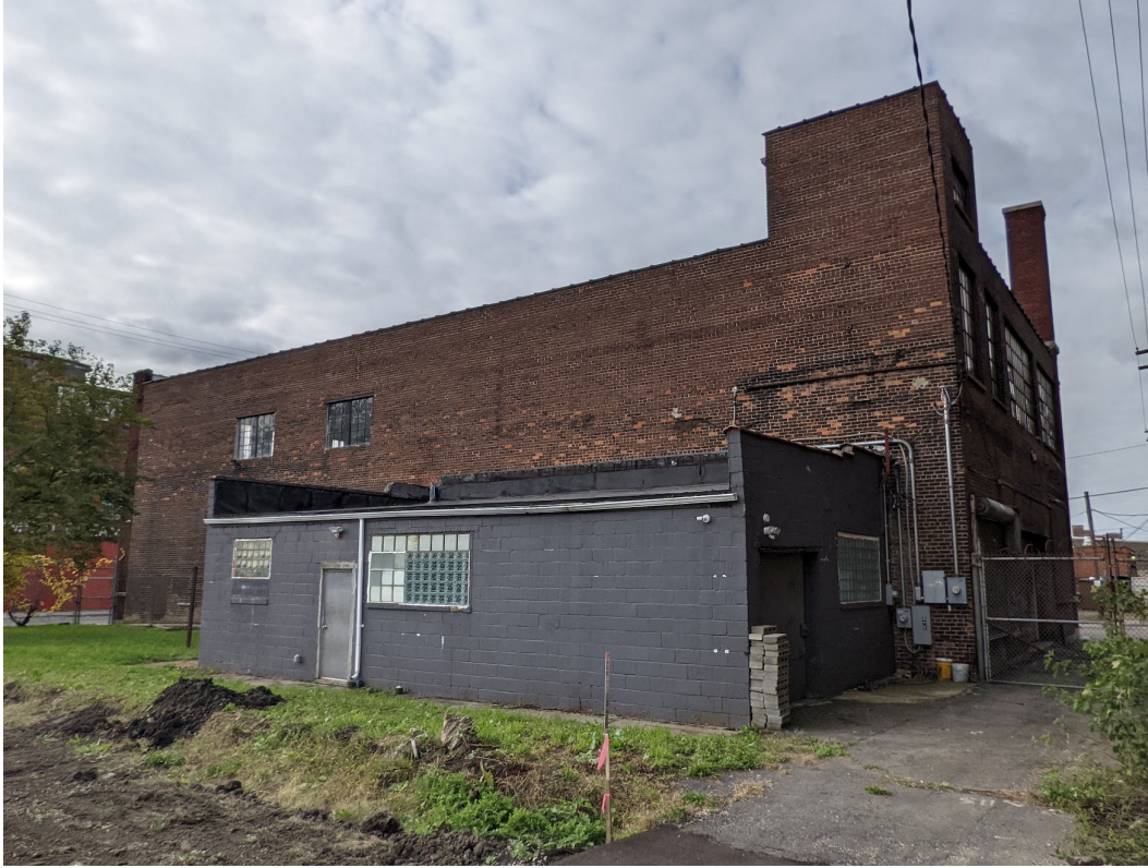
View of secondary east elevation and alley, showing non-contributing concrete block addition. Staff photo, November 2, 2021
