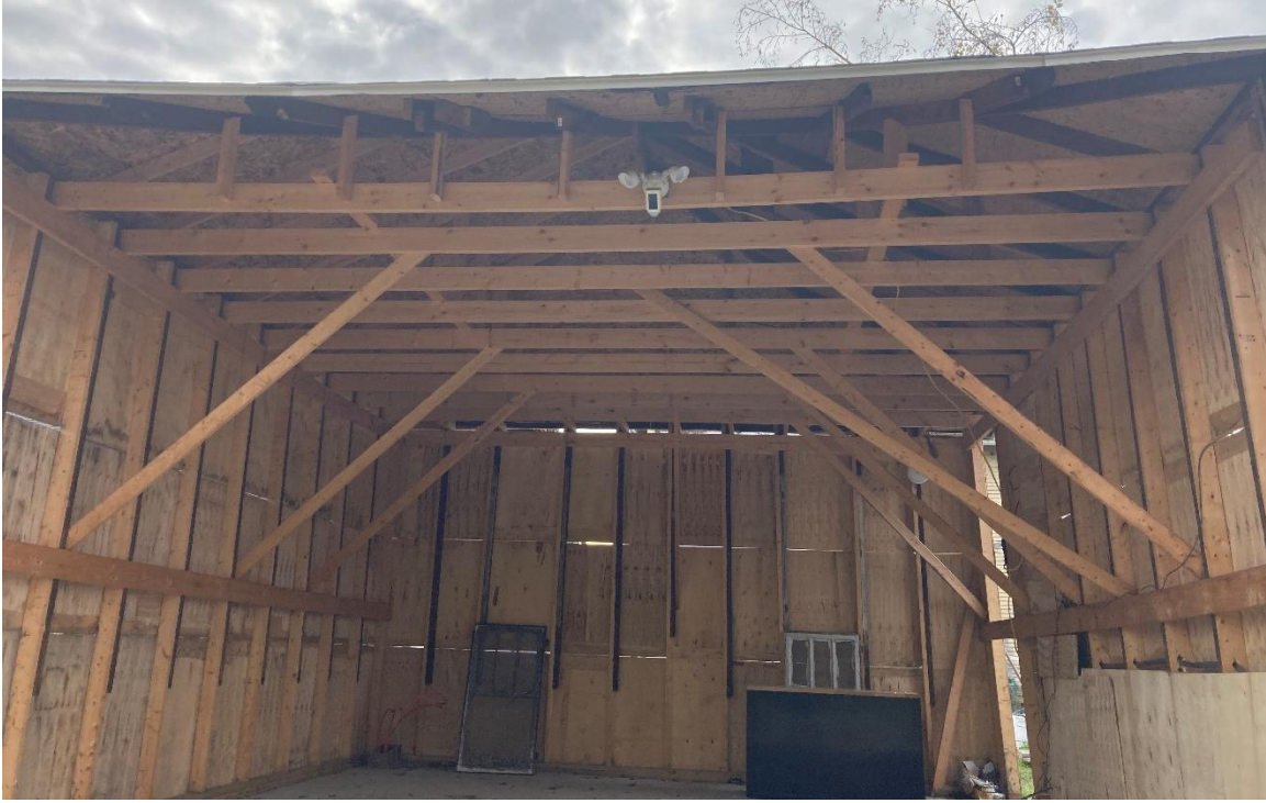
Garage, current appearance
