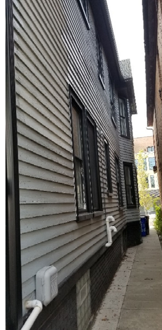
East Elevation (view towards North)
