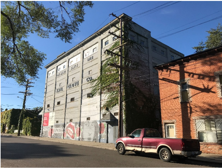
East elevation and portion of north elevation.
