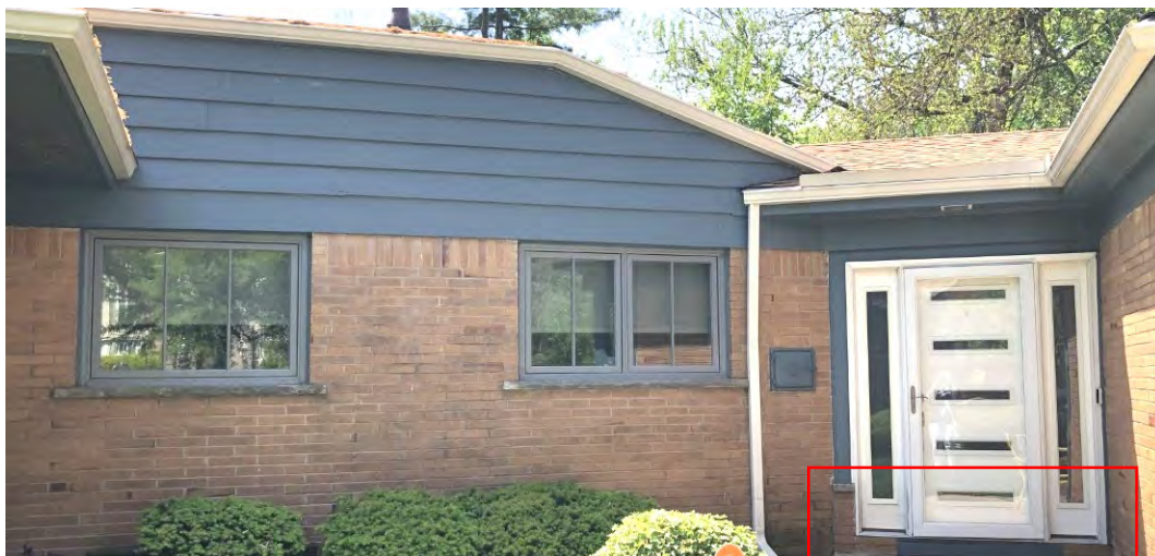
Pella replacement windows and replacement door with sidelights. (HDC staff photo, May 20, 2021). Note the replacement door doesn't fully fill the original door opening.
