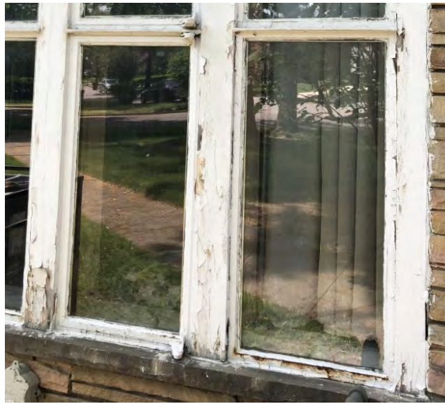
Existing mullions at 19355 Parkside display minimal detailing in keeping with the mid-century design of the house. The width of the wood mullion, in relation to the thinness of the steel sash, is a character-defining detail.
