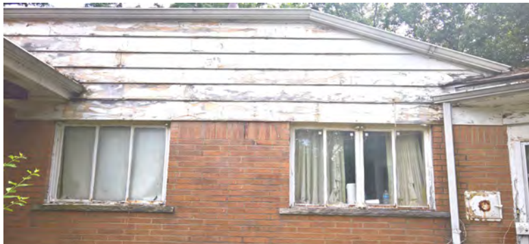
Original steel-framed window sash (casement/fix operation).
