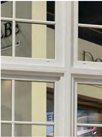
Factory-made mullions are thicker than muntins but often pale in comparison to the dimensionality of historic mullions.
