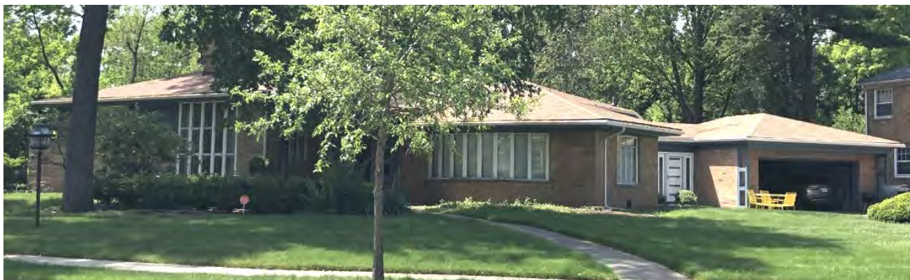
Looking northwest from Parkside at front and east elevation. HDC staff photo, May 20, 2021 (HDC photos on following two pages).
