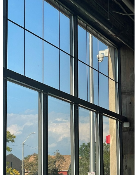
Site Photo 2, by Staff Sept. 17, 2021: Interior (North) front side.
