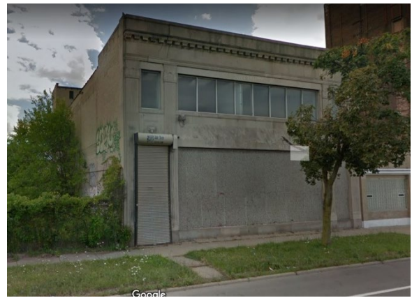
Site Photo 2 by Google Street View 2015: (Northeast) front/side.
