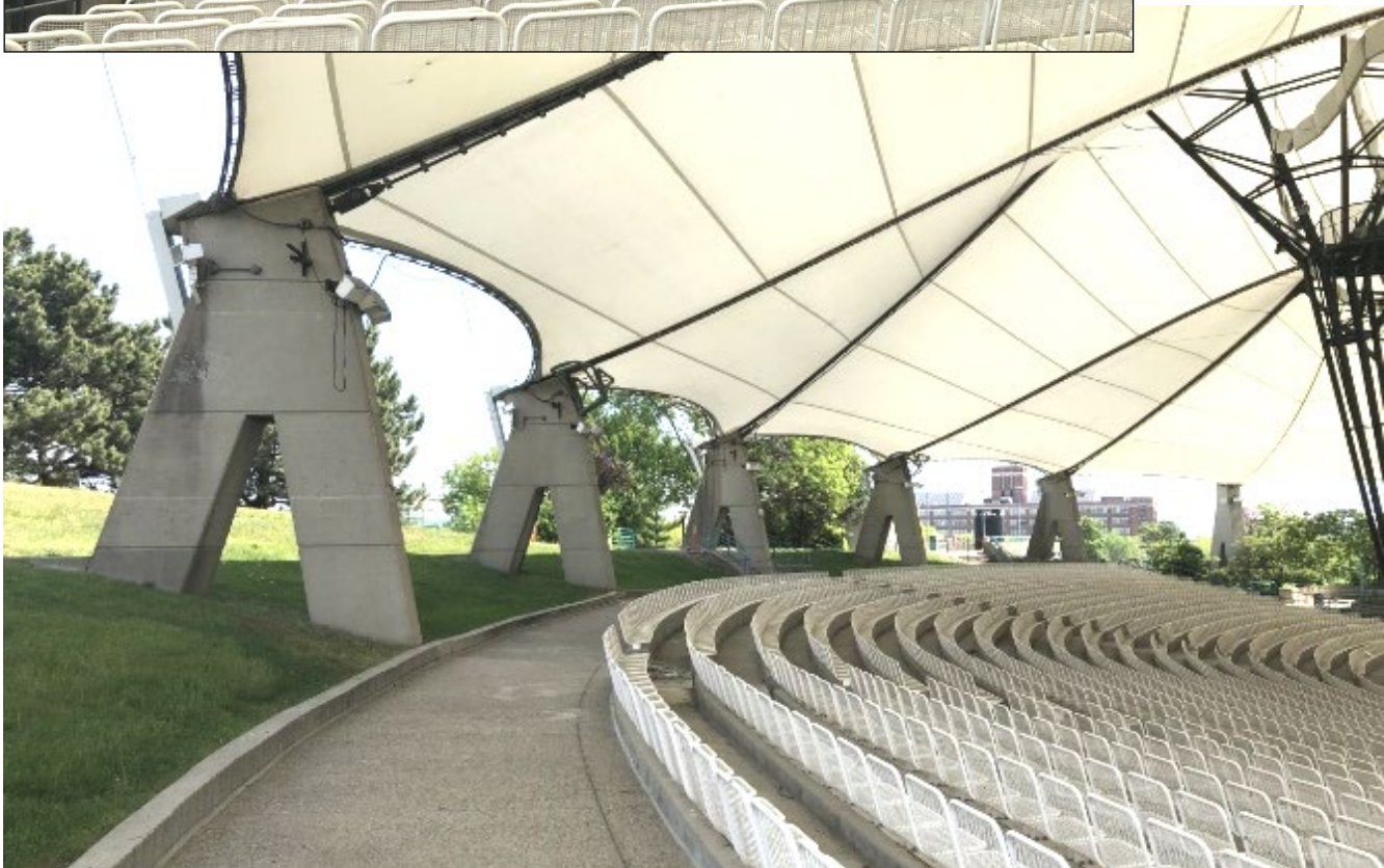
Upper path, looking east. HDC staff photo, May 2021
