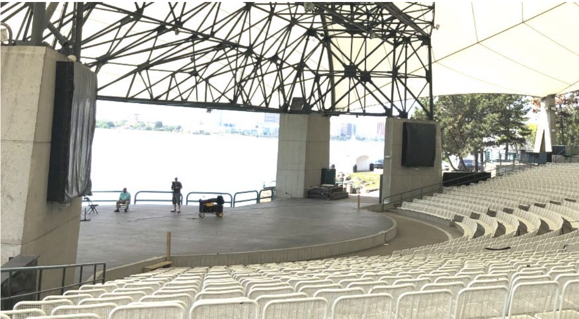
Looking southwest toward stage. Existing signs/ screens flank the stage.
