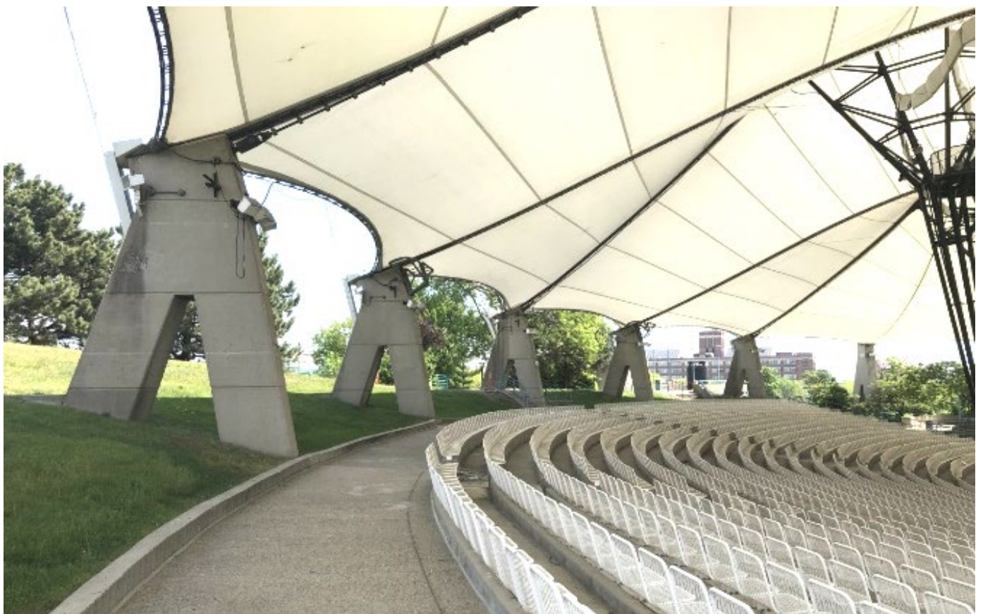
View of the same supports looking toward the east
