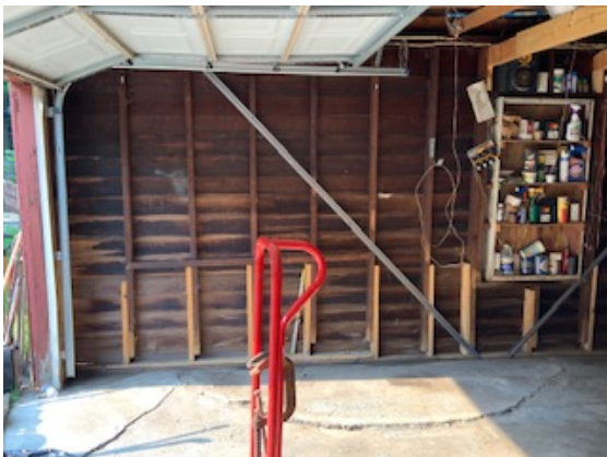
Site Photo 3, by applicant: garage interior
