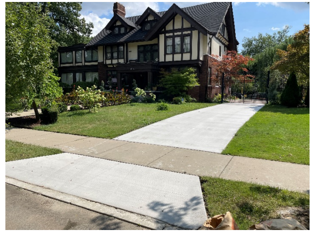
Site Photo 2 by Staff August 31, 2021: Driveway (North) front yard.
