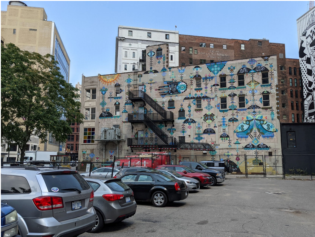
View of the west-facing non-primary, non-character defining elevation (excluding the single character-defining bay at extreme left). Staff photo, July 28, 2021.
