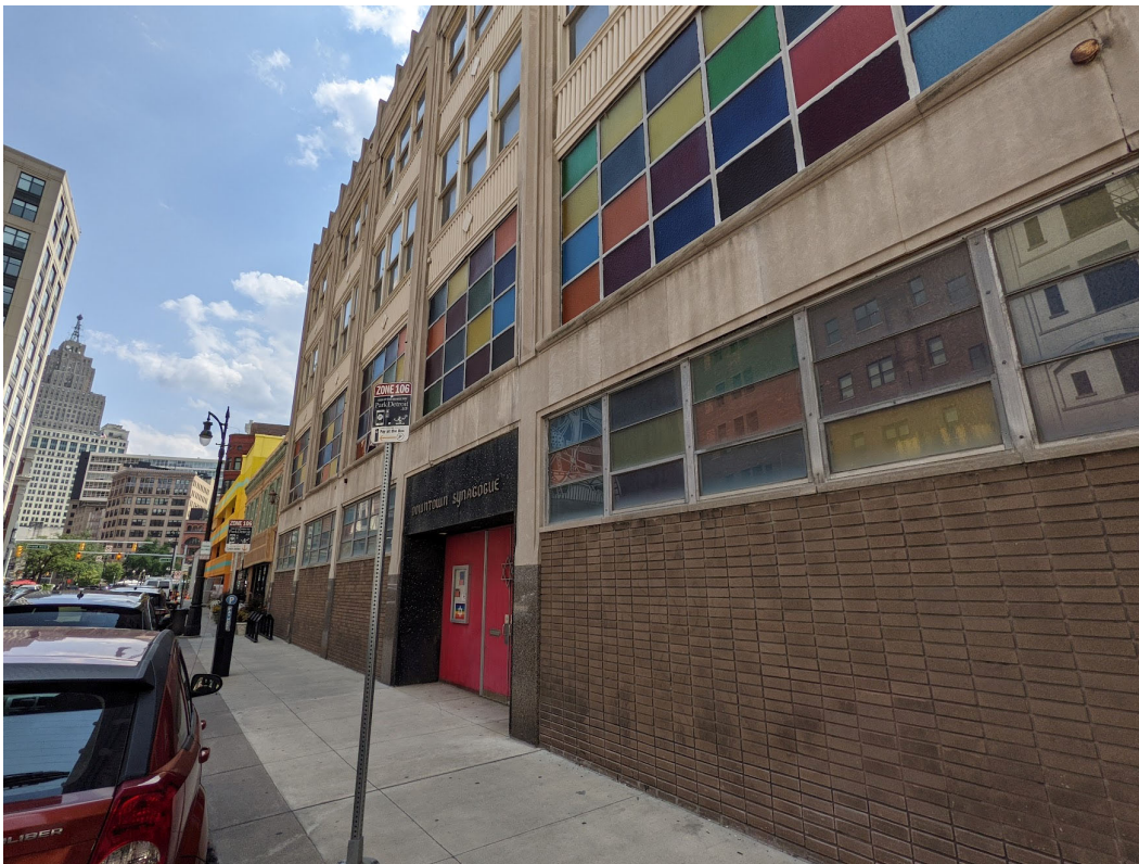
Street-level view of existing conditions at primary (Griswold) elevation, view towards south. Staff photo, July 28, 2021.
