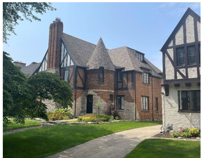
Site Photo 2 by Staff February 7, 2021: (Southeast) side/front elevations.
