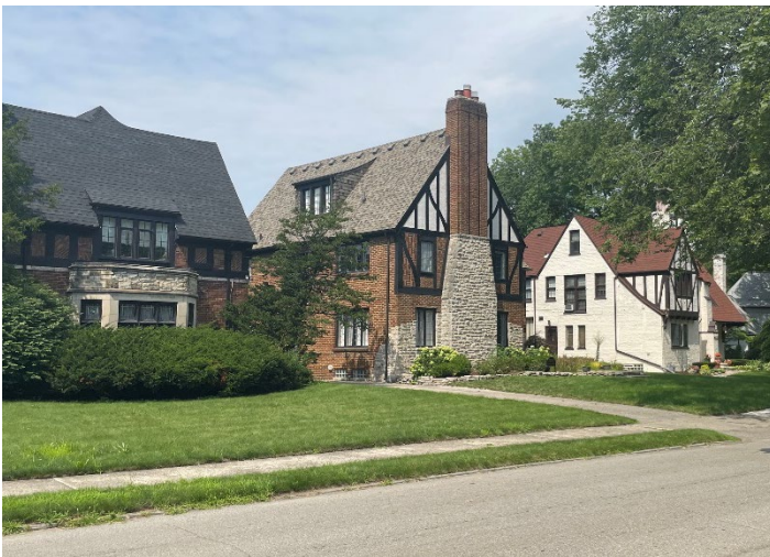
Site Photo 1, by Staff July 22, 2021: (Southwest) side/front elevations.
