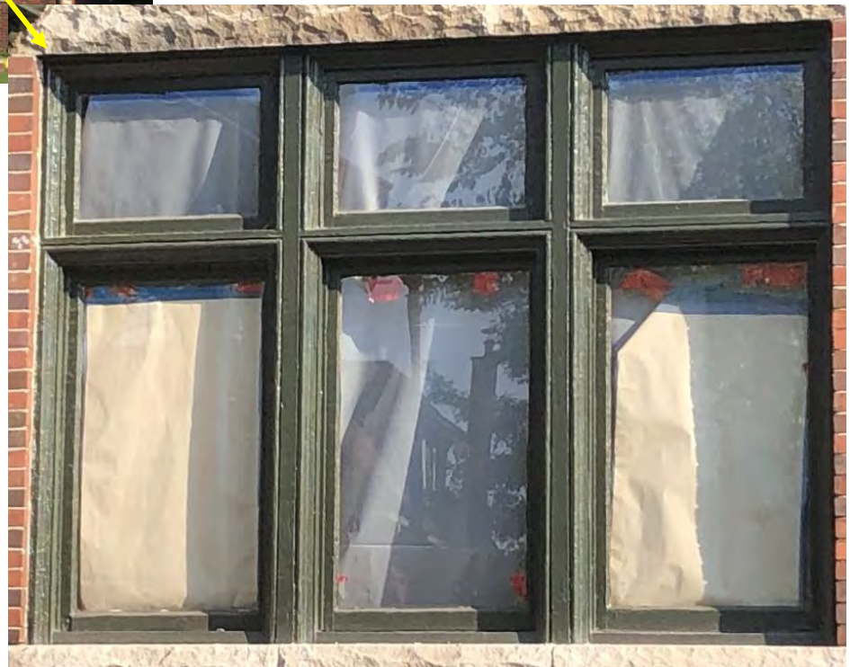
Front elevation, HDC staff photo Close-ups show replacement windows in second floor box bay, and historic sash remaining in first floor openings.
