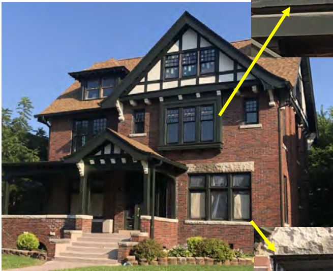
Front elevation, HDC staff photo Close-ups show replacement windows in second floor box bay, and historic sash remaining in first floor openings.
