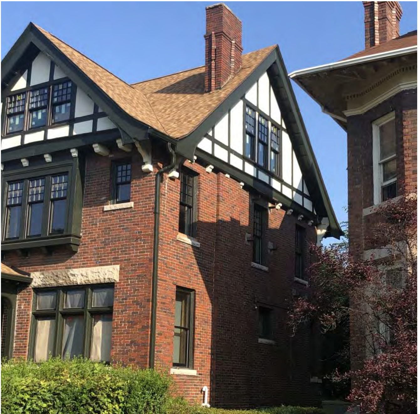
East Elevation, HDC staff photo
