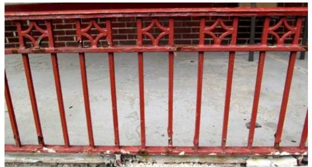
Existing conditions at porch railing. Applicant photo.
