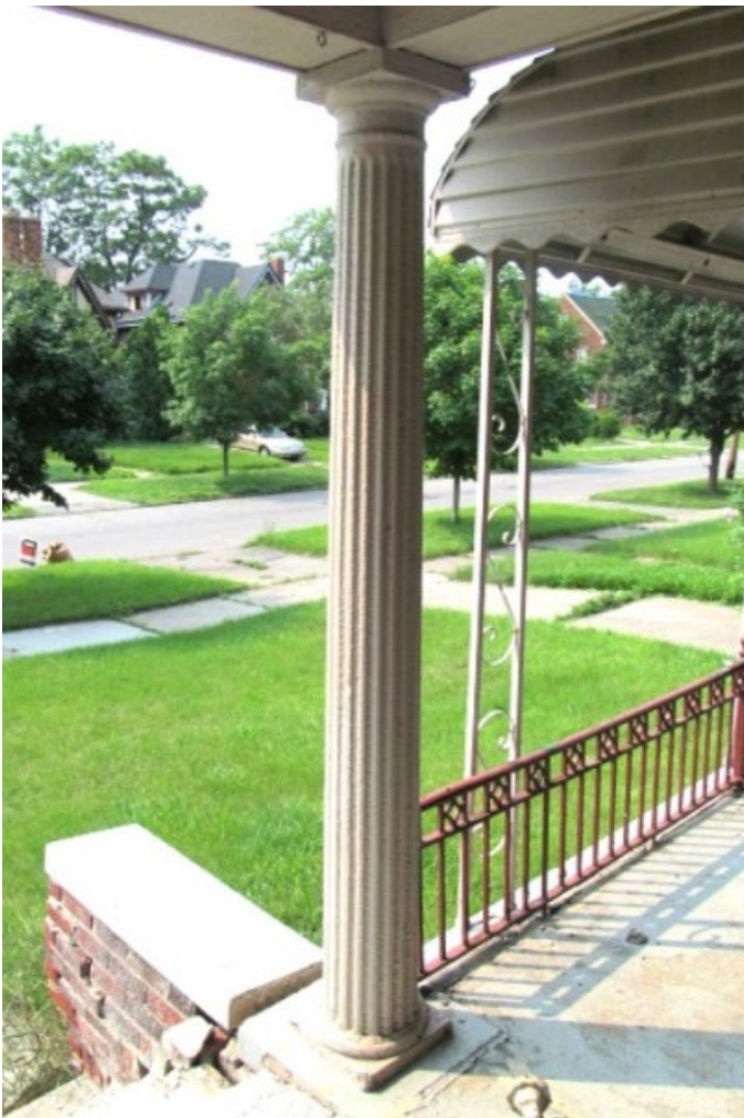
Existing conditions at west (left side) porch column. Applicant photo.
