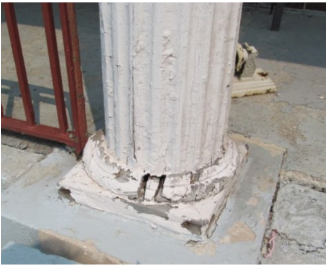
Existing conditions at west (left side) porch column. Applicant photos.
