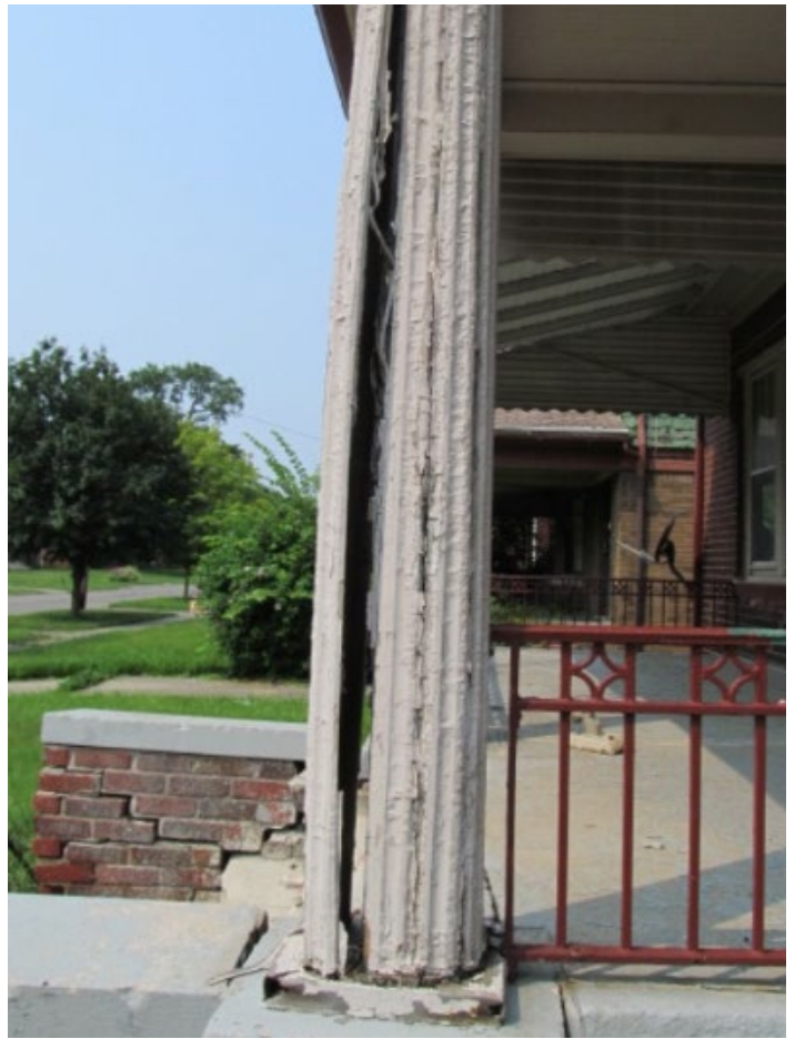
Existing conditions at west (right side) porch column. Applicant photo.
