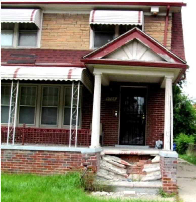
Existing conditions at porch columns and railing. Applicant photo.
