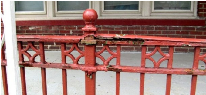
Existing conditions at porch railing. Applicant photo.
