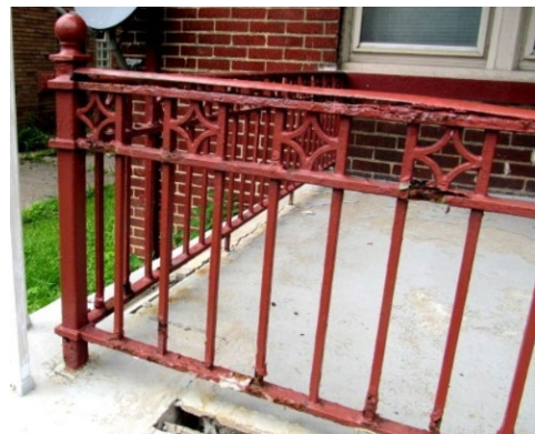
Existing conditions at porch railing. Applicant photo.
