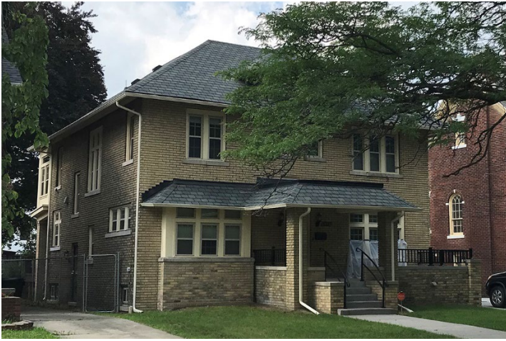
1476 Chicago. View from Chicago Boulevard looking northeast. Photo taken by HDC staff, July 28, 2021.
