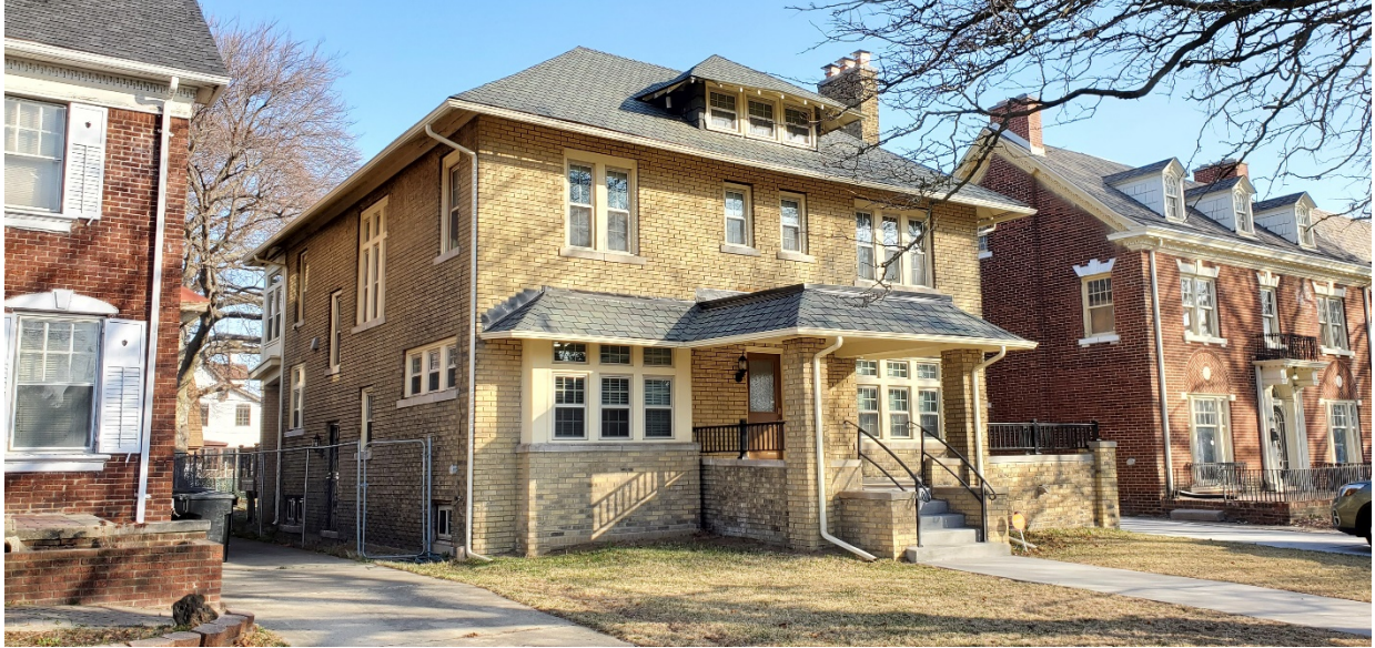
FRONT AND WEST SIDE Existing Residence
