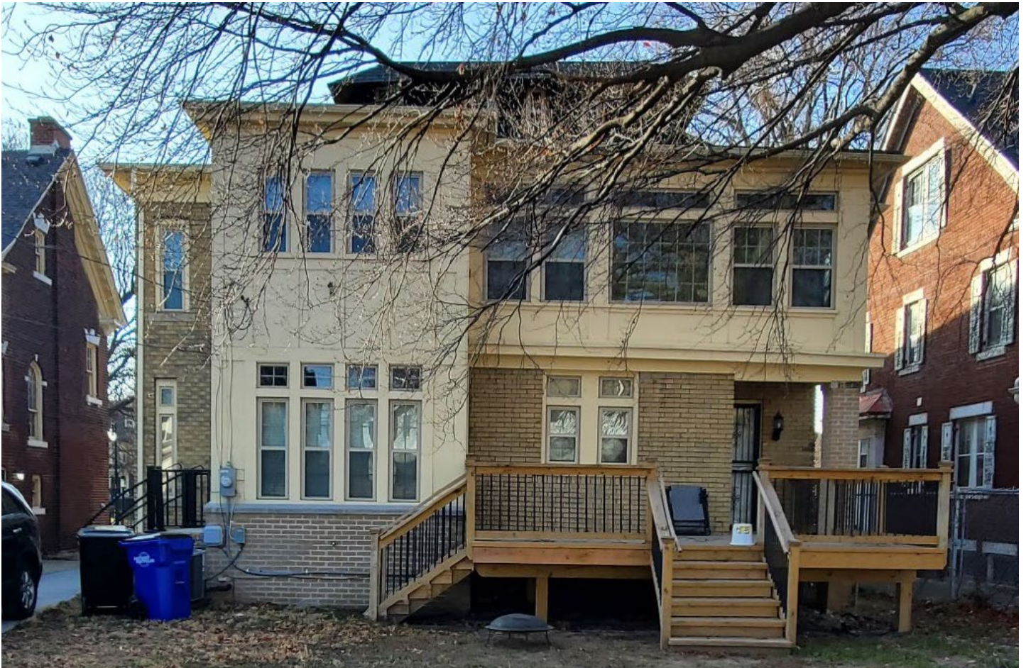
1476 Chicago. View of existing conditions at rear, looking south. Applicant photo.
