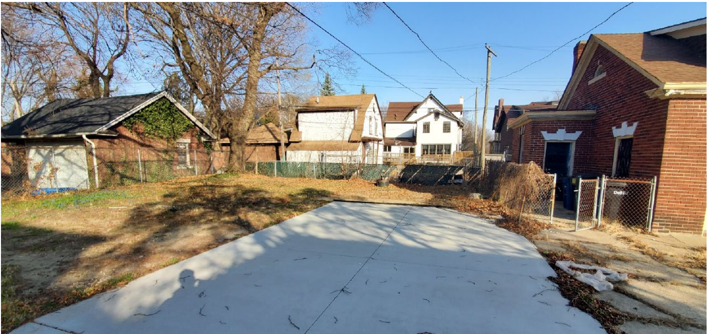
1476 Chicago. View of existing conditions at rear, location of proposed garage, looking north. Applicant photo.
