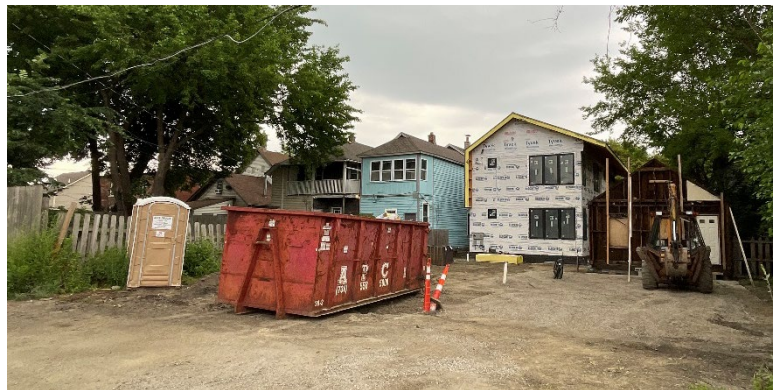
Site Photo 2 by Staff June 25, 2021: Carport site (West) rear.
