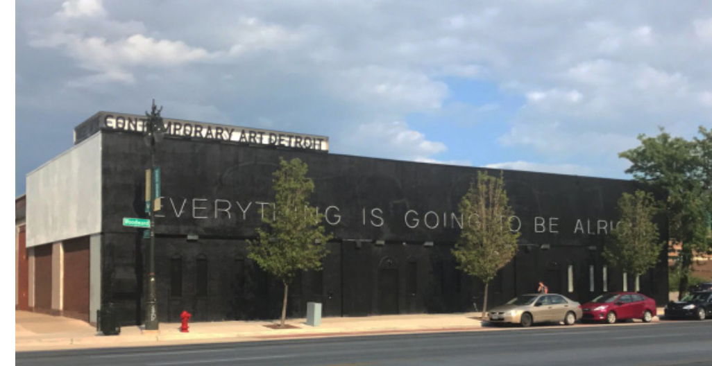
4454 WOODWARD AVE - MUSEUM OF CONTEMPORARY ART DETROIT CIVIC / INSTITUTIONAL (ADJACENT TO SUGAR HILL HISTORIC DISTRICT)
