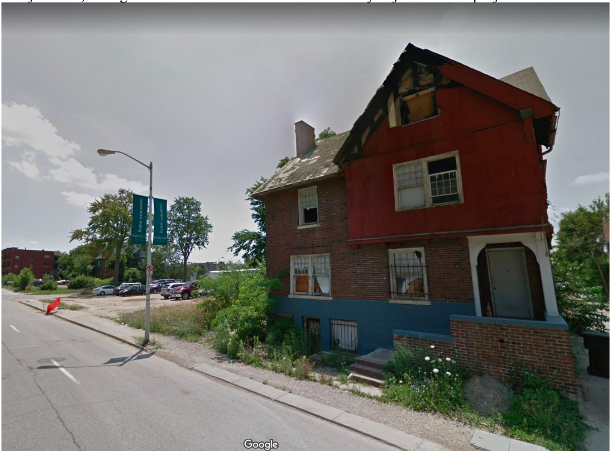
Project area, facing southwest. Note historic house directly adjacent to the project area
