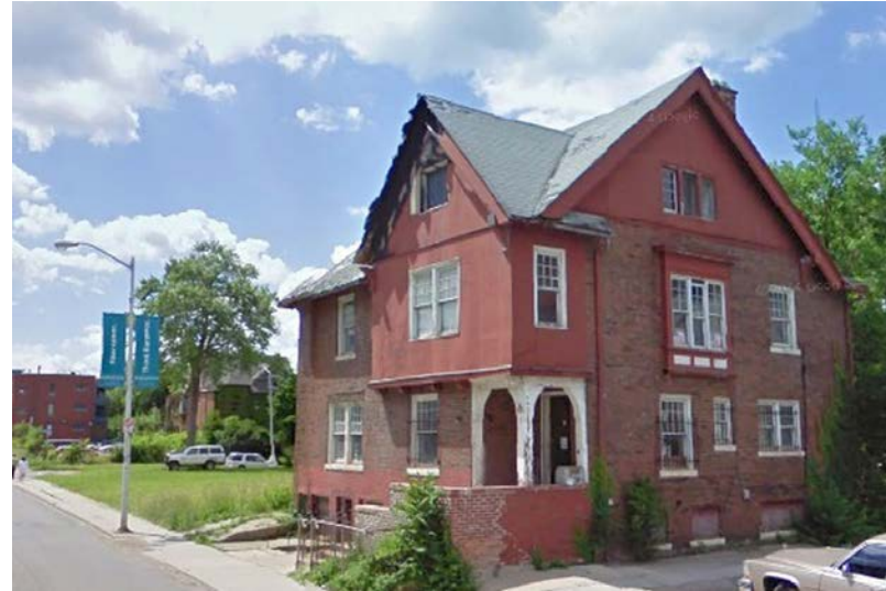
4635 JOHN R ST. - MCCOLLESTER HOUSE VACANT
