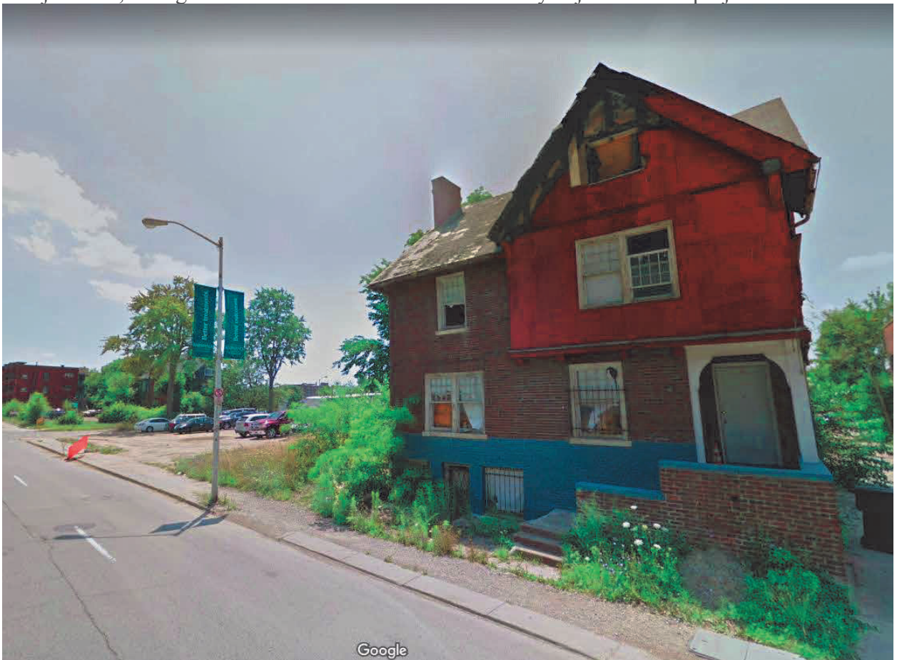
Project area, facing southwest. Note historic house directly adjacent to the project area
