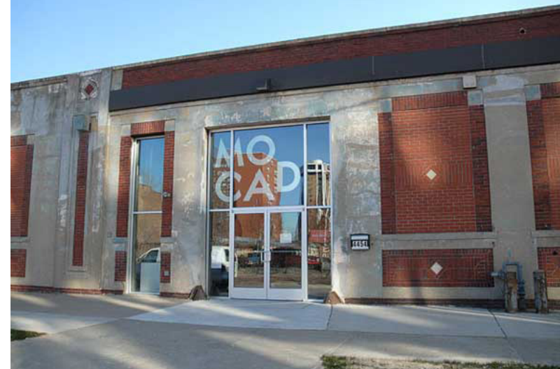
4454 WOODWARD AVE - MUSEUM OF CONTEMPORARY ART DETROIT CIVIC / INSTITUTIONAL (ADJACENT TO SUGAR HILL HISTORIC DISTRICT)
