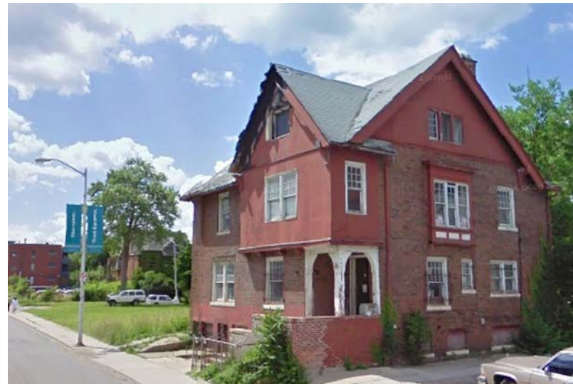
4635 JOHN R ST. - MCCOLLESTER HOUSE VACANT
