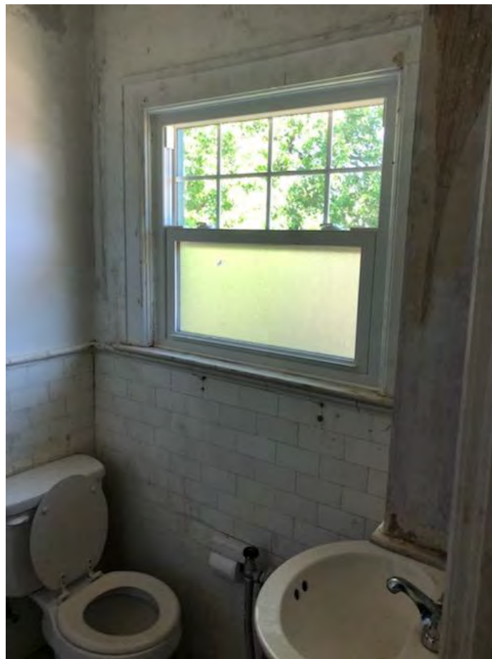
UPPER BATHROOM (BACK BEDROOM)
