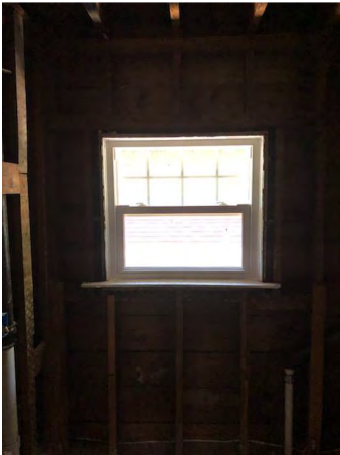
2ND FLOOR BATHROOM (SIDE)
