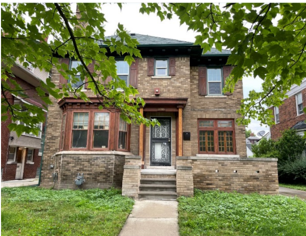
Site Photo 1, by Staff June 25, 2021: (Southeast) front side
