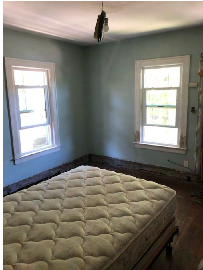
2ND FLOOR BEDROOM (SIDE AND BACK)
