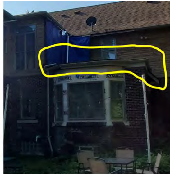
After removal – June 2021
