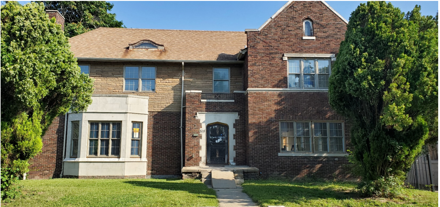
535 Arden Park. View of existing conditions at front facade – windows replaced and metal railing removed without HDC approval. Applicant photo.
