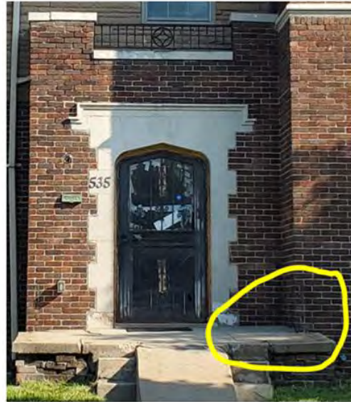
After removal – June 2021
