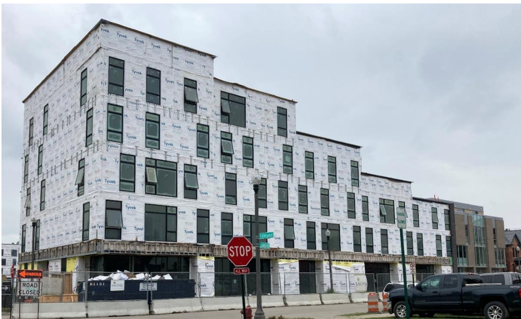
200 Edmund Place, current appearance from the northwest; staff photo, June 2, 2021.
