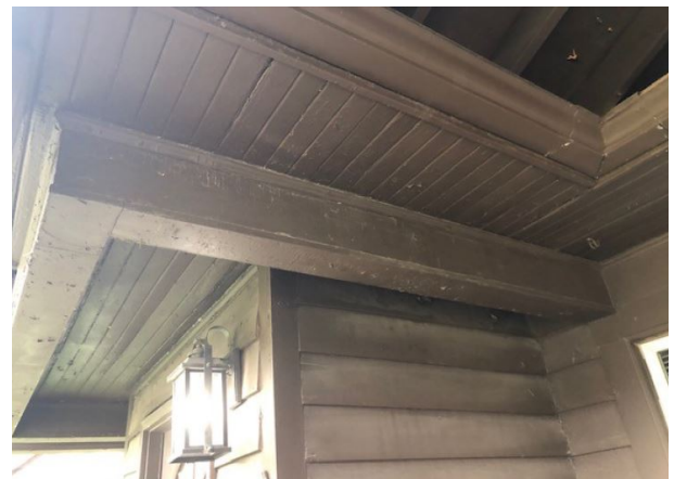
Porch Ceiling Detail 1, by Applicant: original ceiling.
