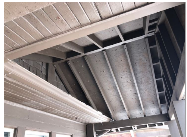
Porch Ceiling Detail 2, by Applicant: original and new ceiling.
