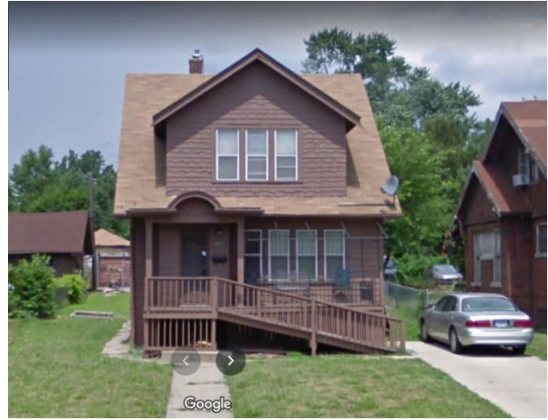
Site Photo 3, by Google July, 2009: (Southeast) front elevation.
