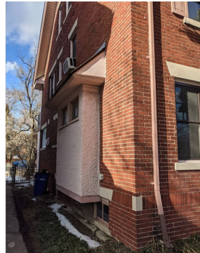
Site Photo 5 by Applicant: (South) side/front, before work complete.
