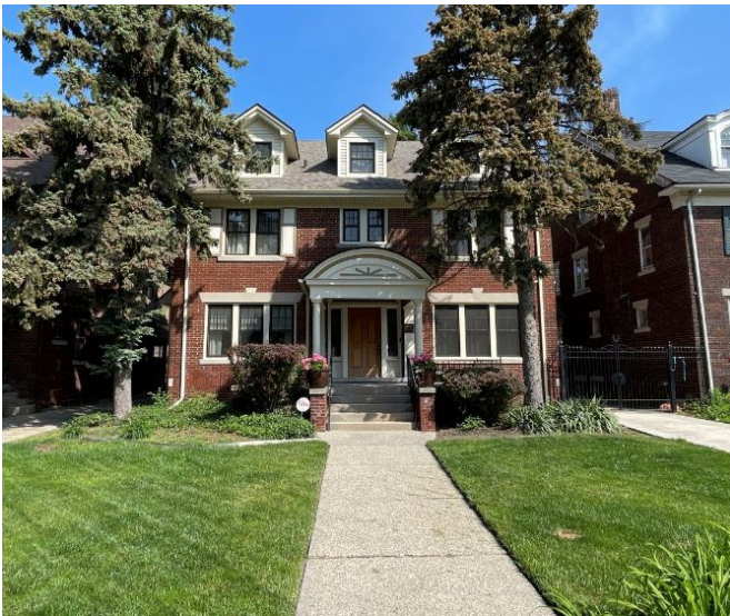
Site Photo 1, by Staff May 21, 2021: (Southeast) front side
