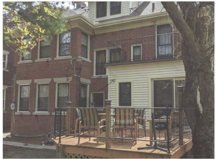
Site Photo 4, by Applicant (northwest) rear, arrows indicate work complete.
