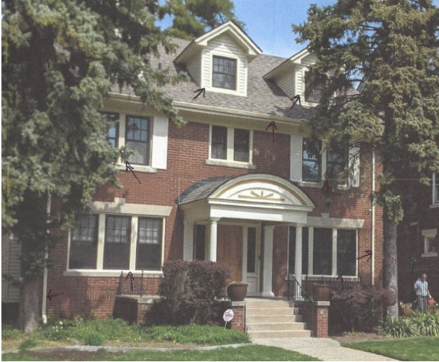
Site Photo 3, by Applicant (Southeast) front, arrows indicate work complete.
