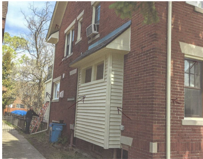
Site Photo 4 by Applicant: (South) side/front, arrows indicate work complete.
