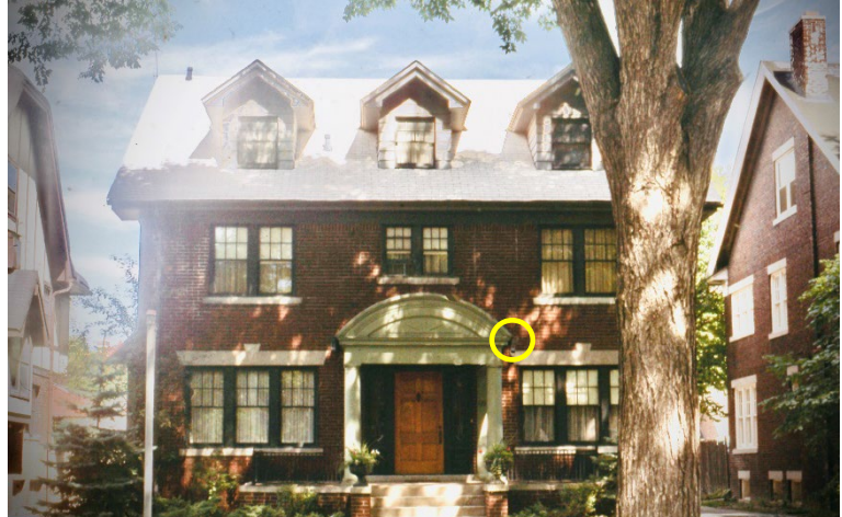
1974 Designation photo: Front elevation, original down spout location.
