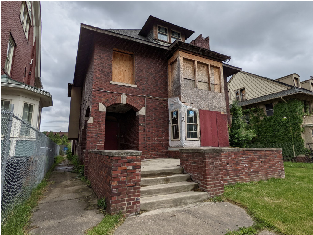
Front view of 240 Mack. Staff photo, May 26, 2021.
