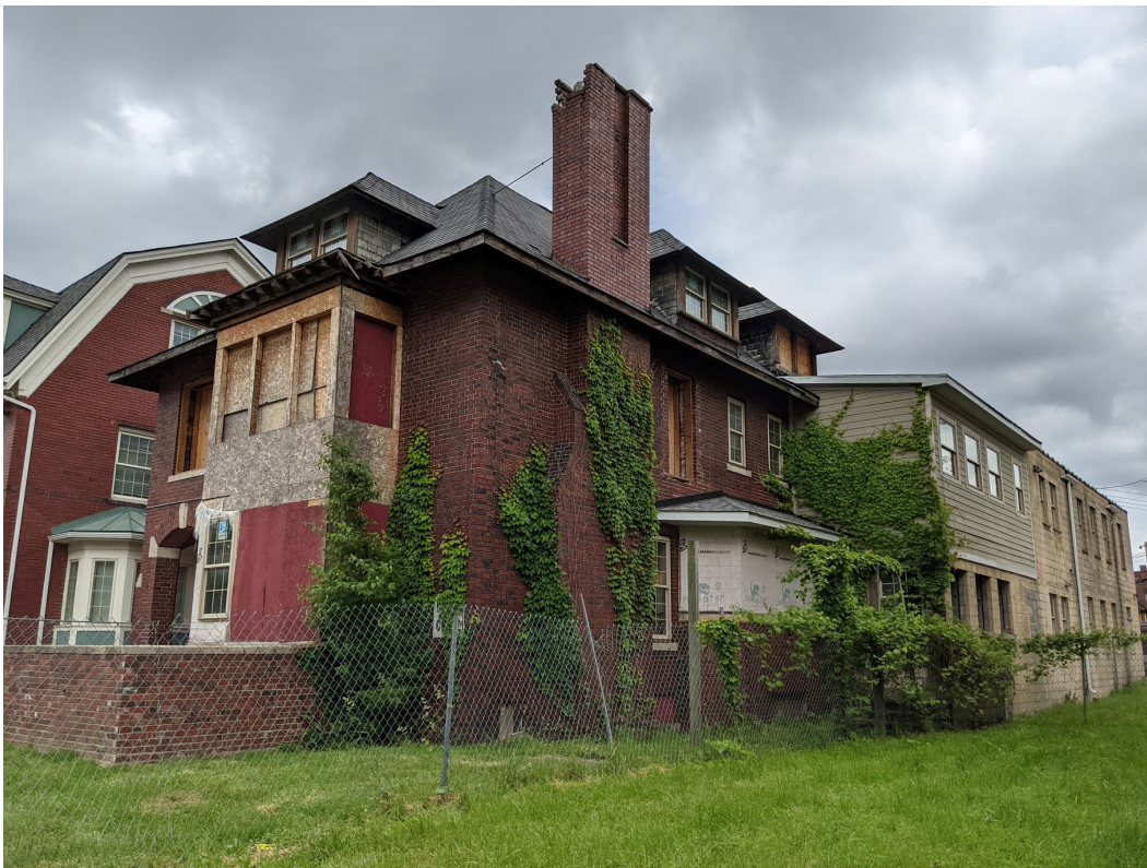
View of 240 Mack to the southeast, as seen from Mack, showing the large, non-historic rear addition towards rear. Staff photo, May 26, 2021.
