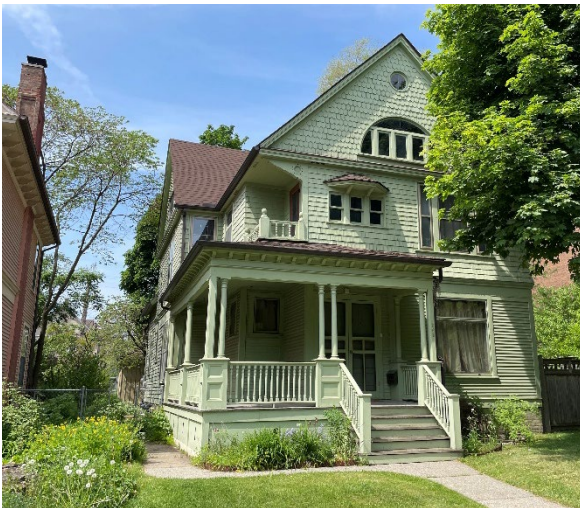
Site Photo 1, by Staff May 21, 2021: (Northeast) front side
