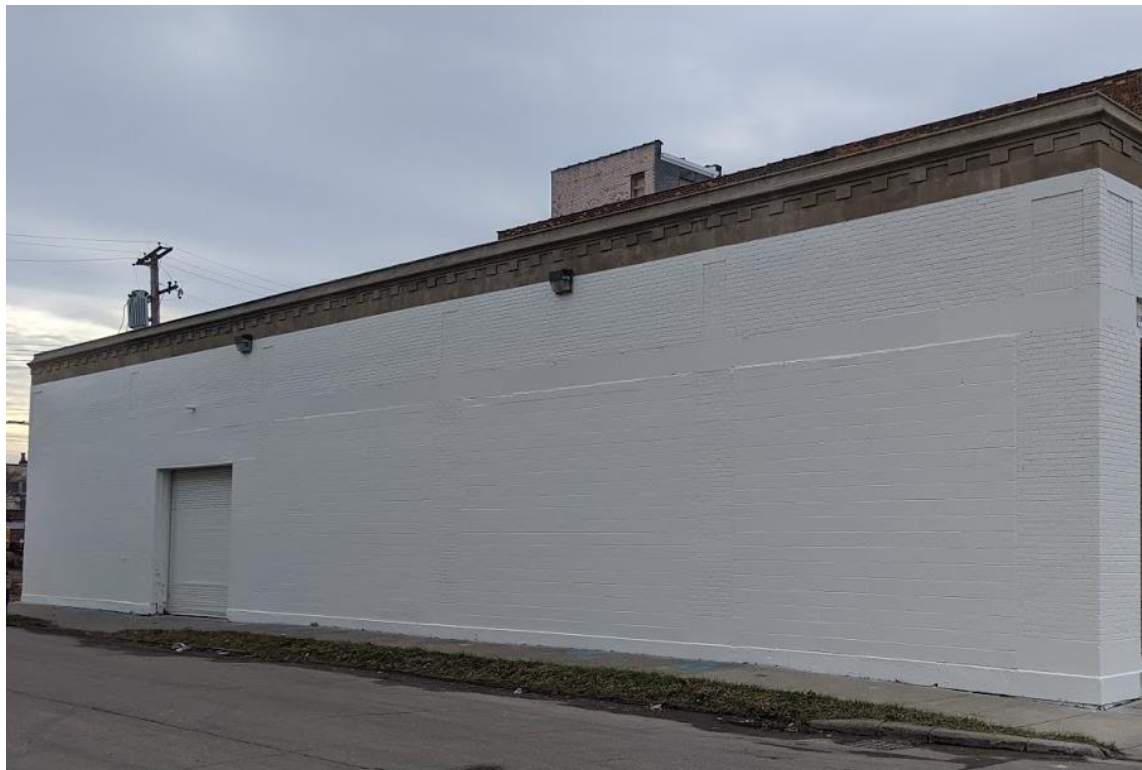
2857 E. Grand, side/east elevation, showing the project area/proposed location of the proposed door opening infill, 5/1/2021
