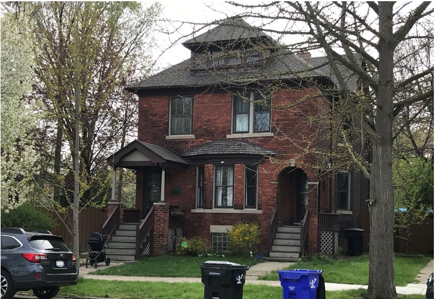
4217 Lincoln. View from Lincoln Street looking southwest. Photo taken by HDC staff, April 23, 2021.
