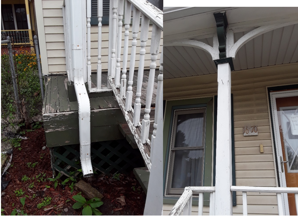
The corner of the porch rail will go to the corner of the porch floor.
