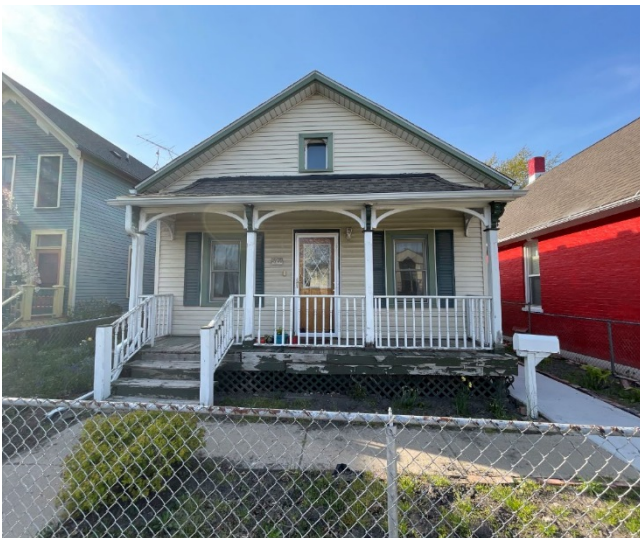
Site Photo 1, by Staff April 27, 2021: (Sout) front side
