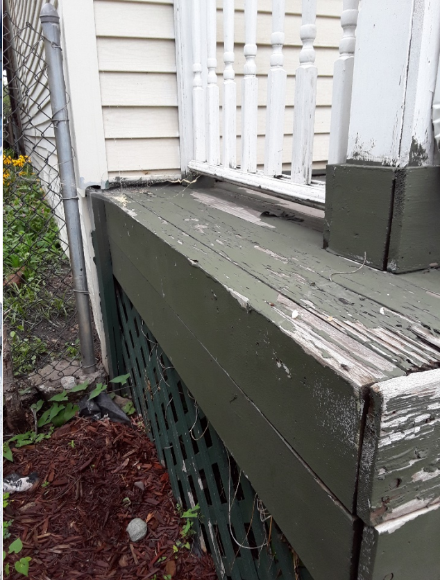
West side of porch.
