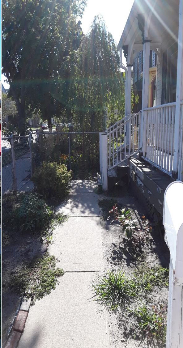
Paint peeling from front bottom fence
