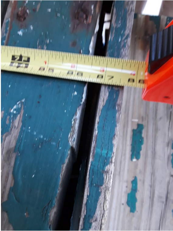
End of porch floor is at 87 ½ inches long.
