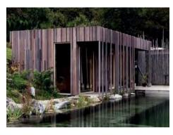
öko skin flex 125 mm, various colours, vertical installation, screwed on wooden substructure
