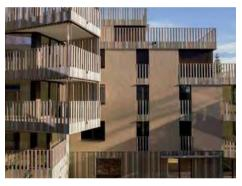
öko skin flex 147 mm, various colours, vertical installation, rivets on aluminum substructure
