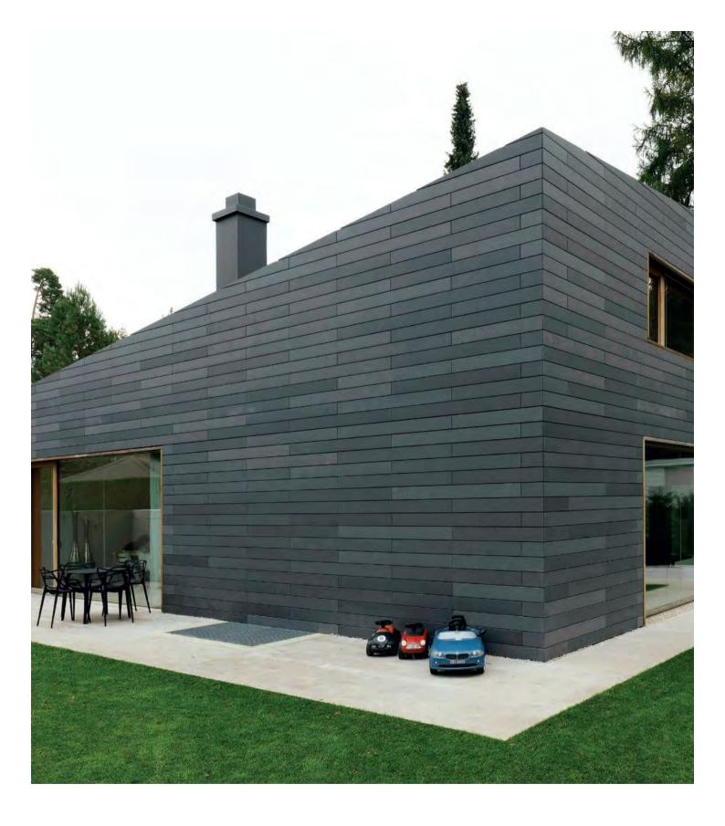
**öko skin** slat wall panels made of glassfibre reinforced concrete
