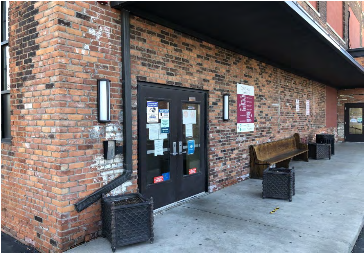
5716 MI AVE, West Elevation Entrance-Close UP
