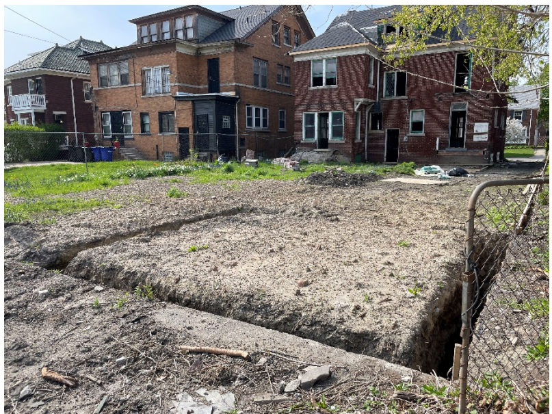
Site Photo 2 by Staff April 27, 2021: Garage site (Southeast) side/rear.
