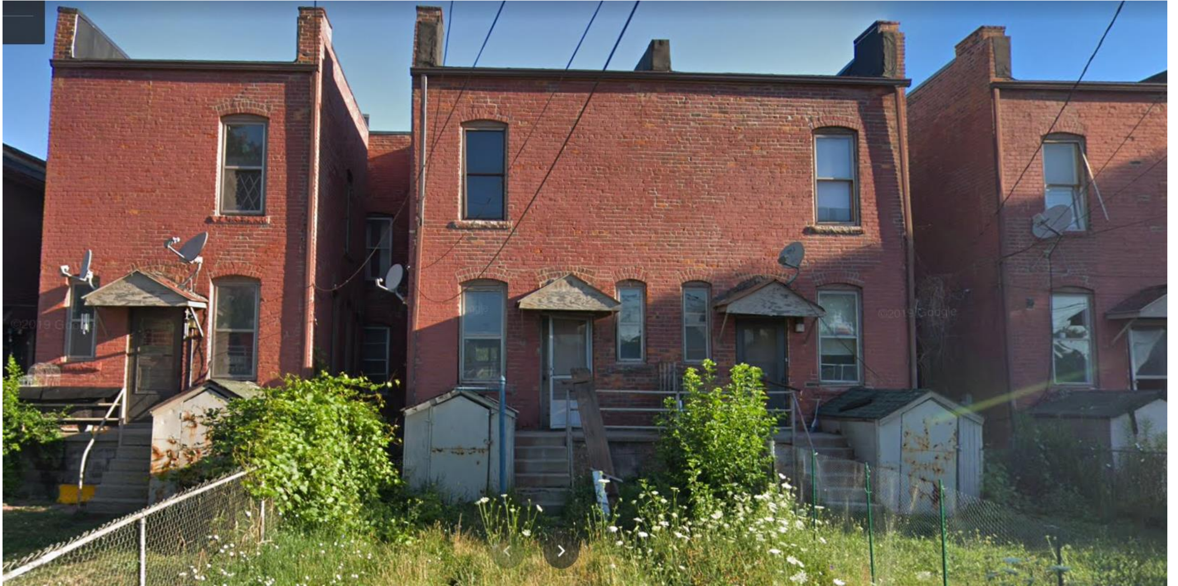
Rear elevations, prior to unapproved work
