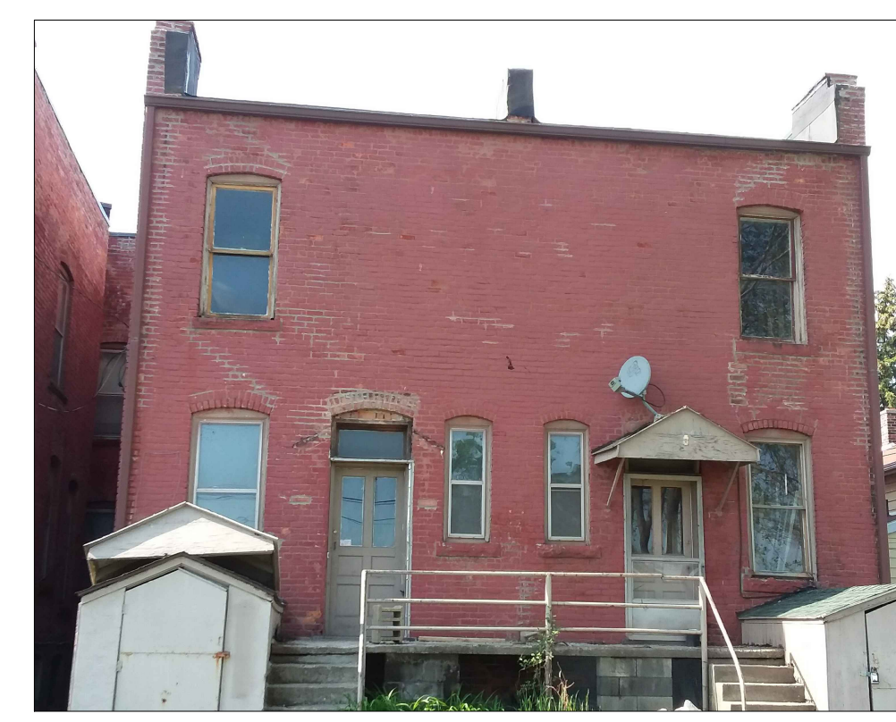
Building Before Renovations South Wall - Units 1 and 2
