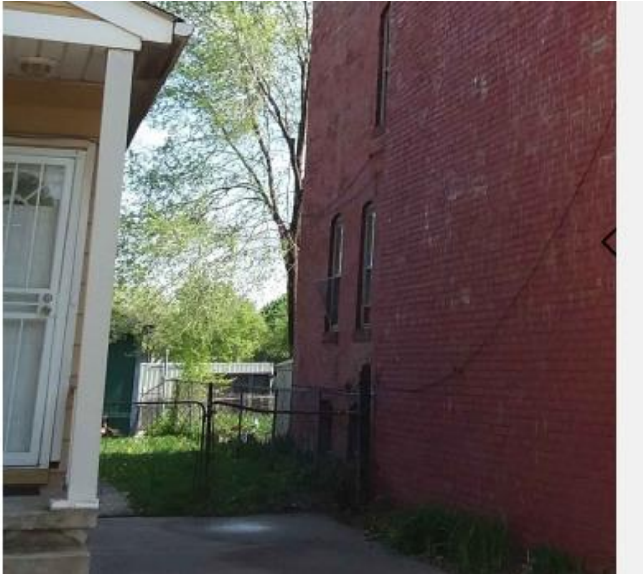
Side elevation, prior to unapproved work. Note painted brick
