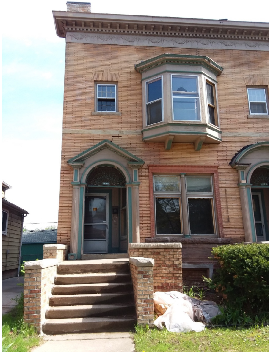
General View Existing Front Wall Before Start of Repairs
