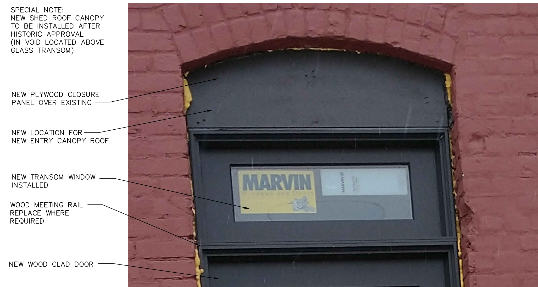
Enlarged View of New Door Transom Opening
