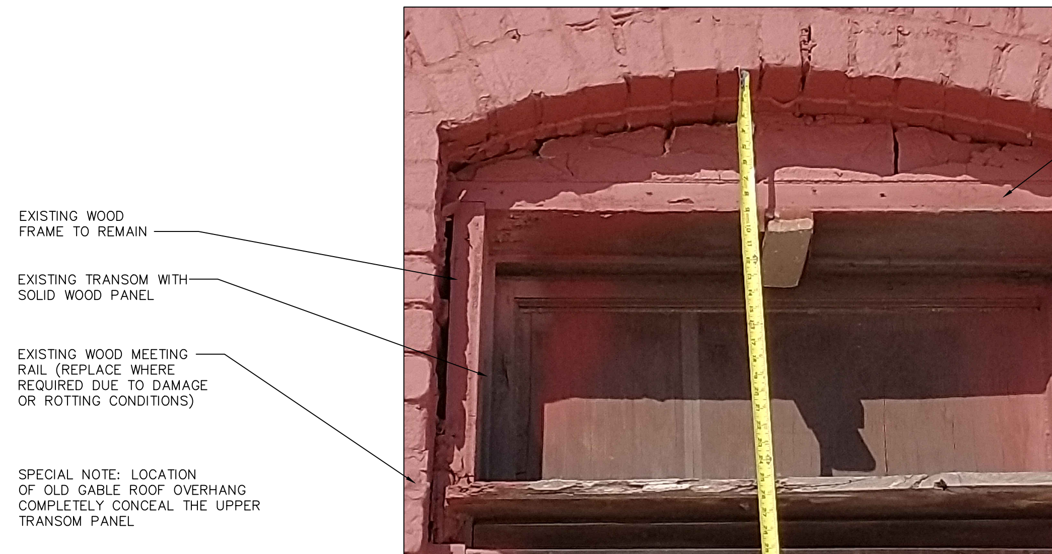
Enlarged View of Existing Door Transom Opening
