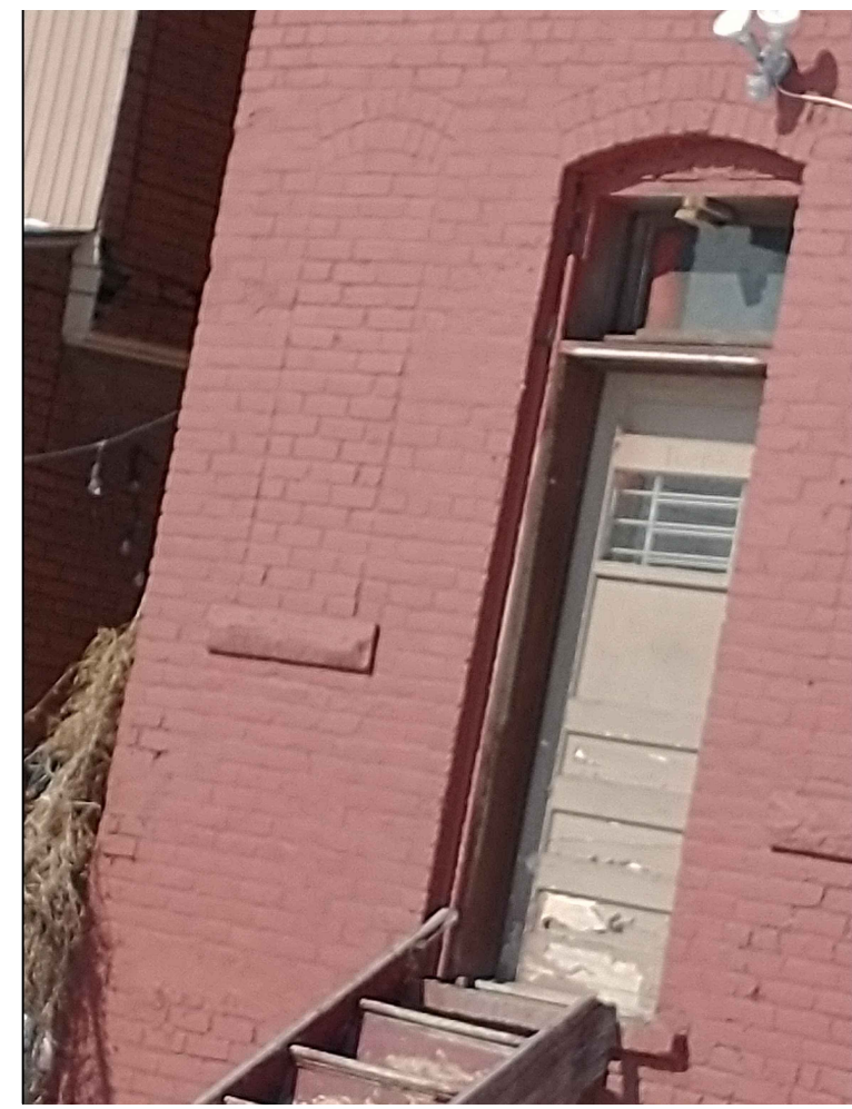
Existing Unit Rear Door (CURRENT)
