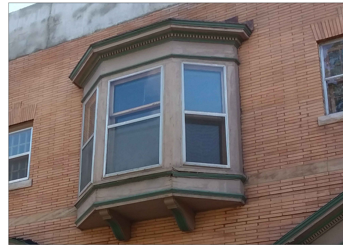
Bay Window Before Replacement
