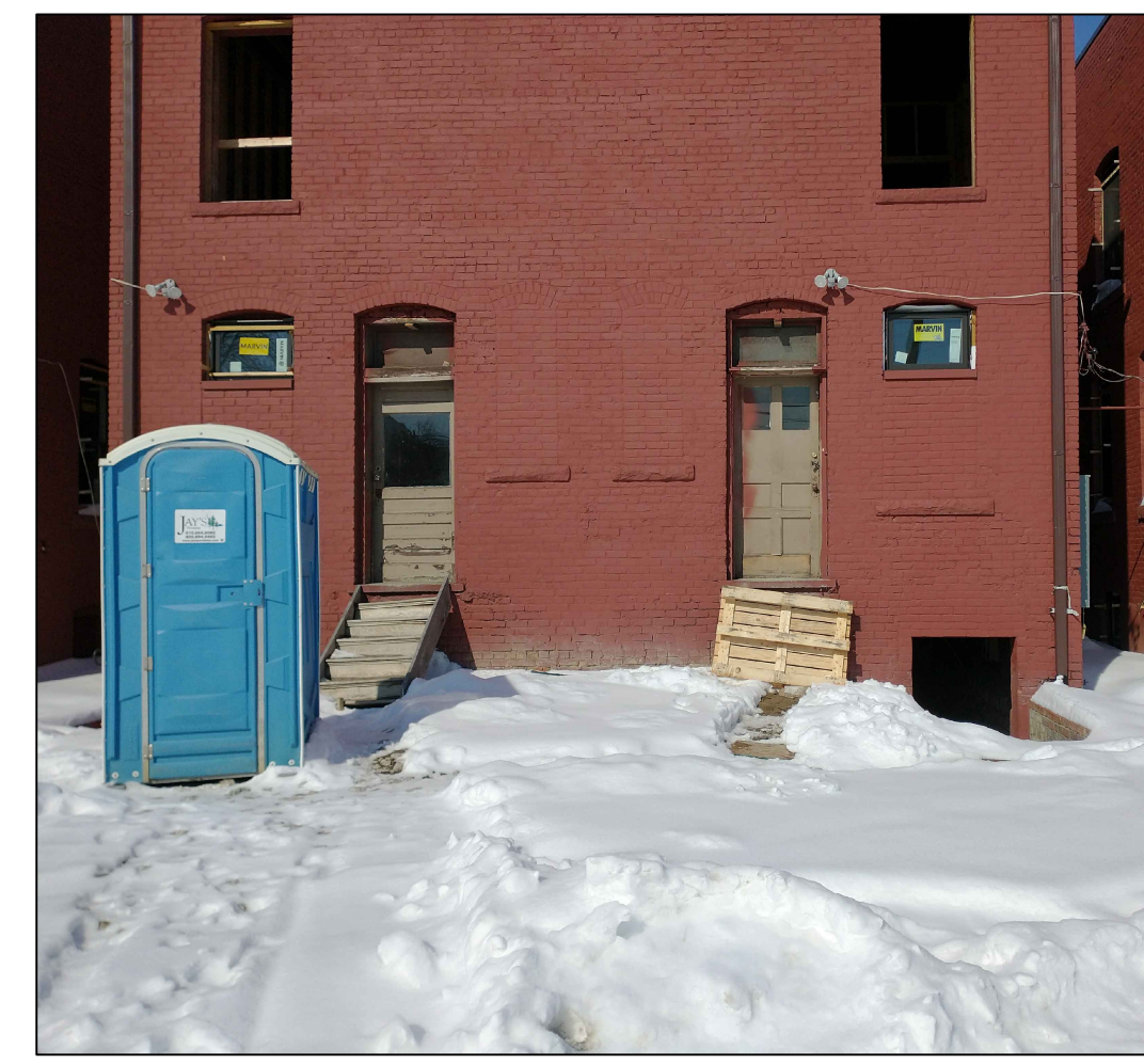
Existing Unit Rear Door (CURRENT)
