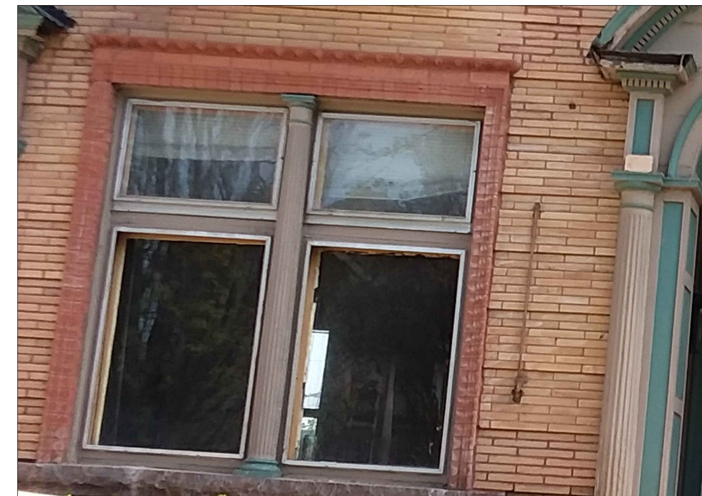
Window Before Replacement
