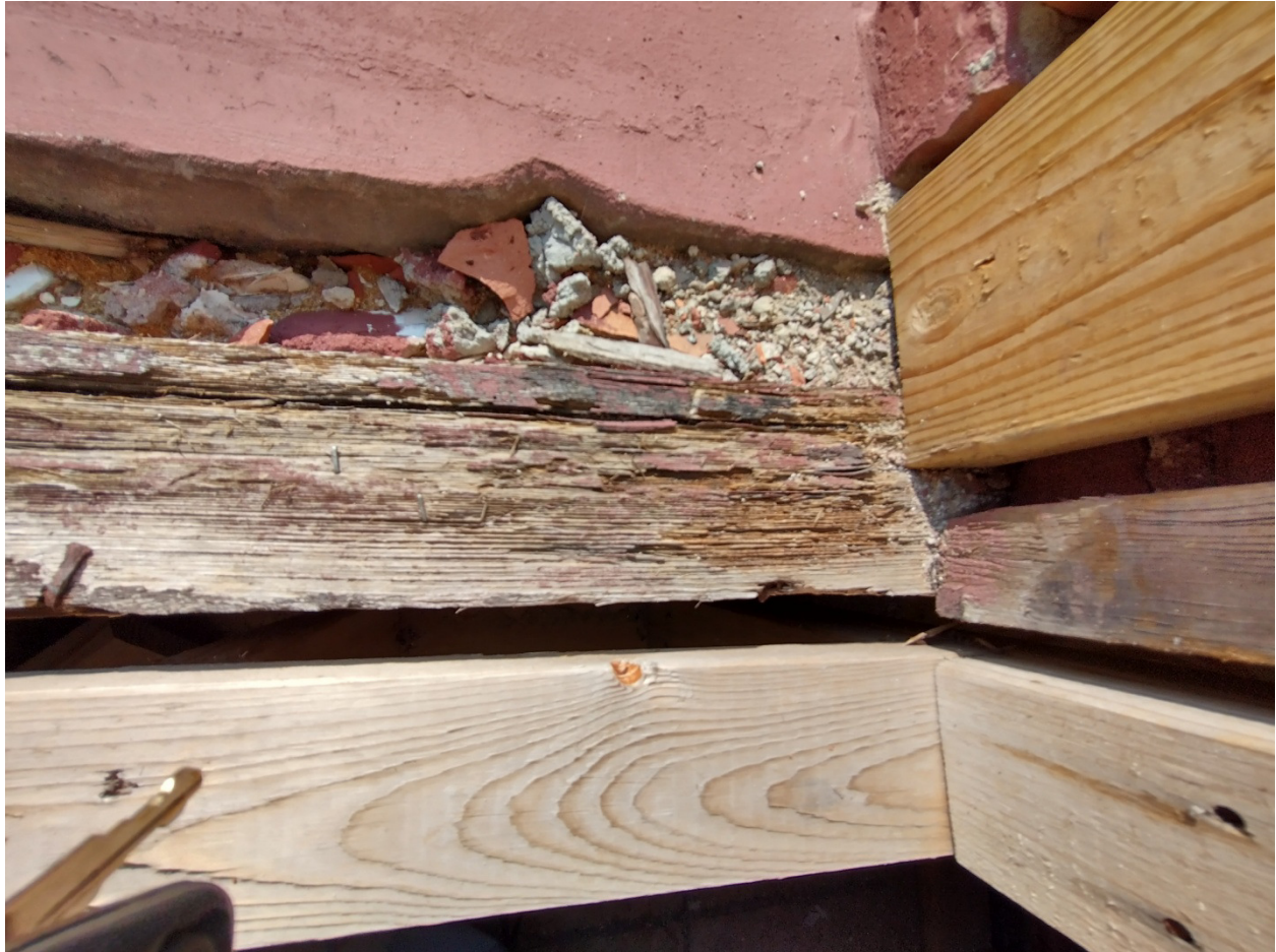
Typical Wall Cavity View
