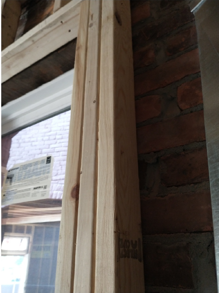
View of New Interior Framing @ exterior wall
