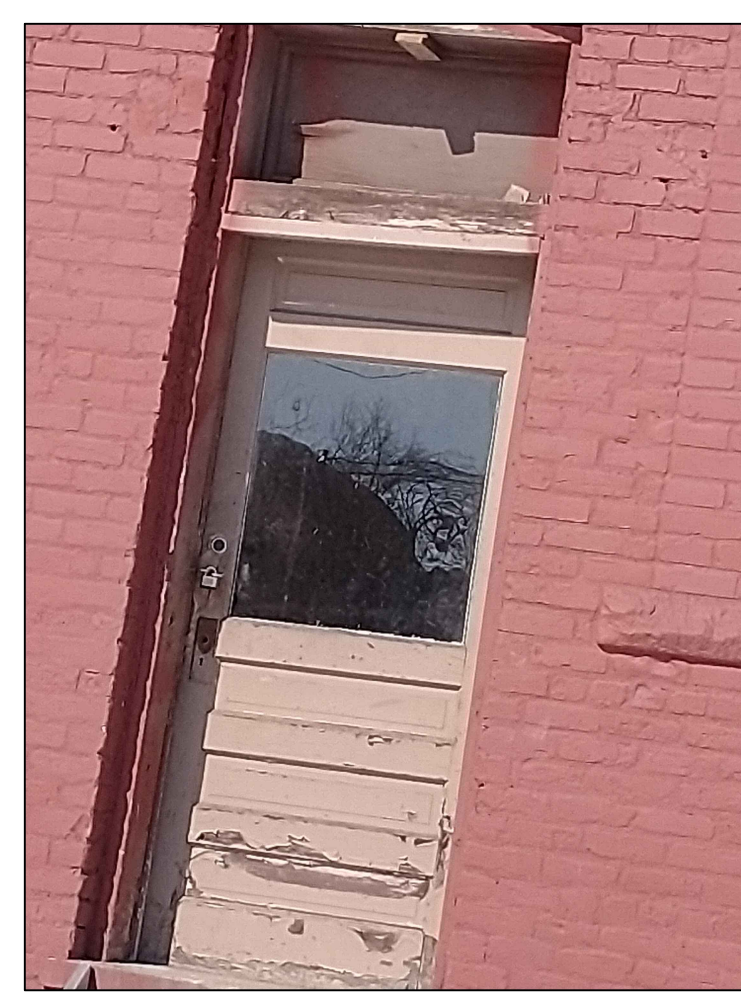
Existing Unit Rear Door (CURRENT)
