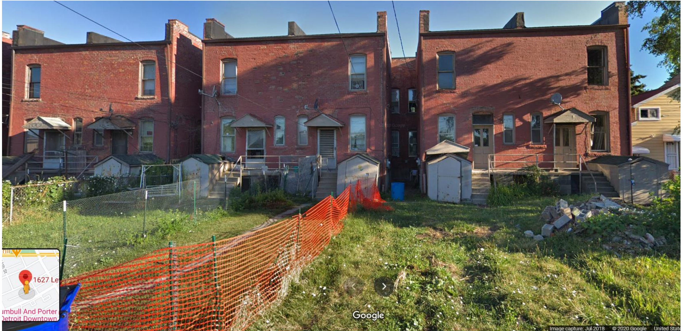
Rear elevations, prior to unapproved work
