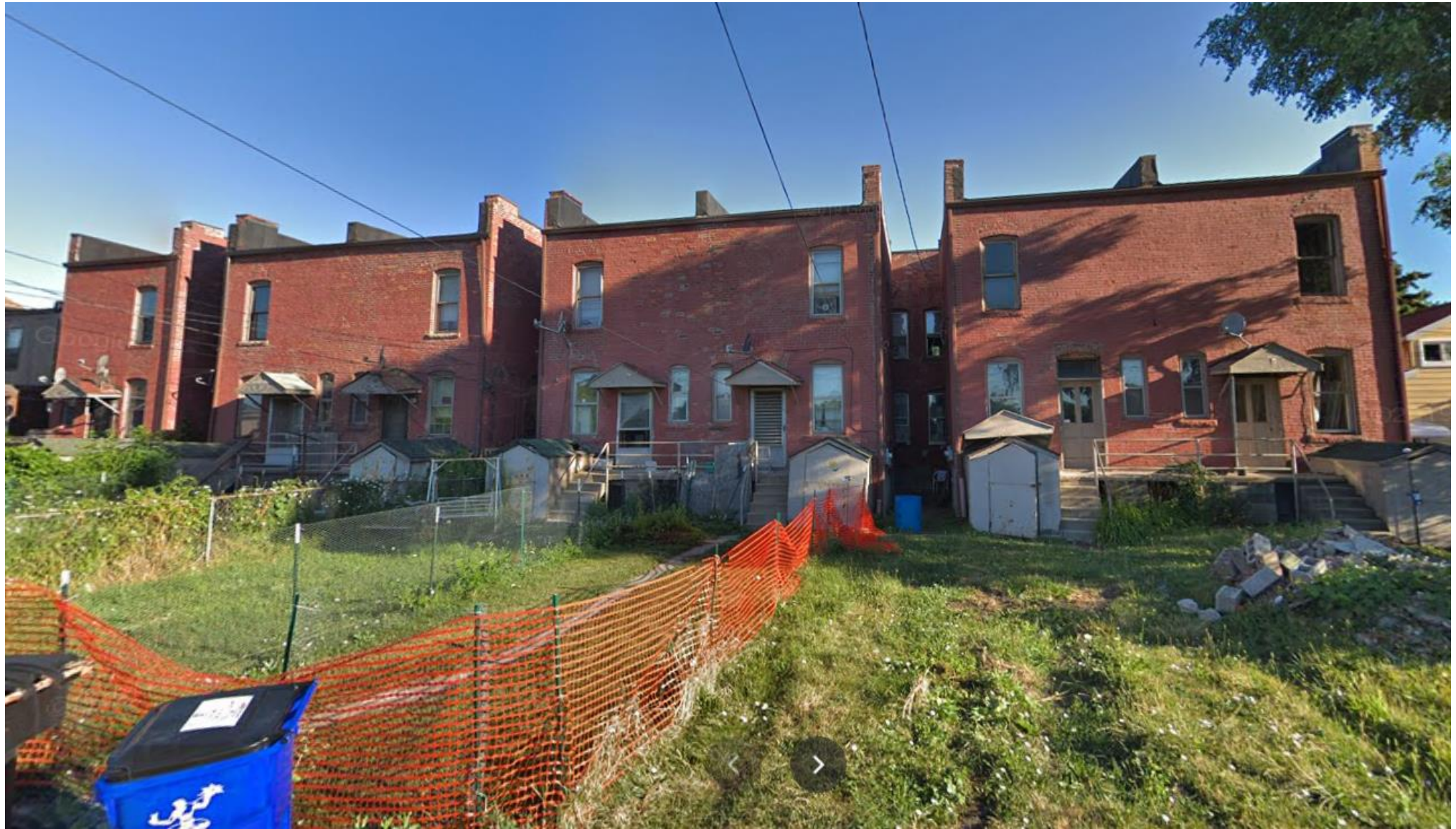
Rear elevations, prior to unapproved work
