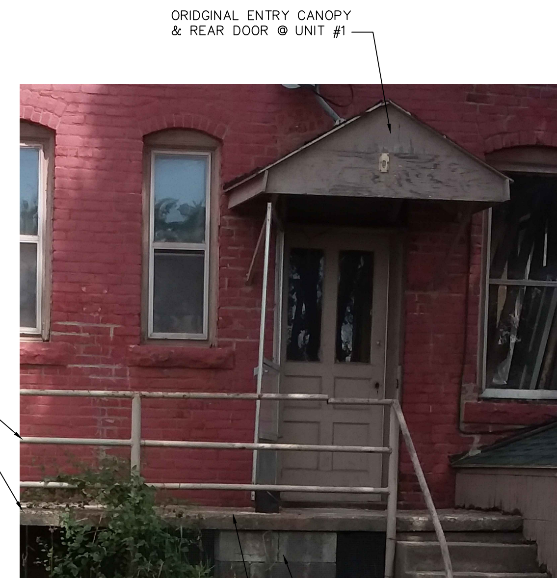
Existing Porch - Rear Door
