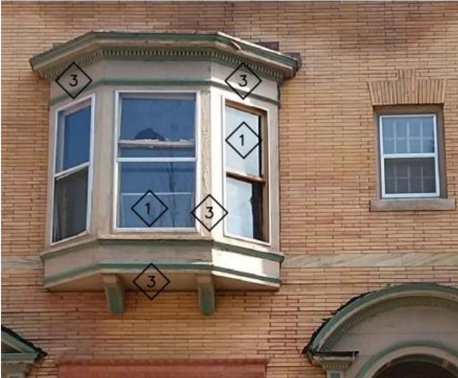
Second-story bay window (typical) prior to unapproved work, note 1/1/ windows. Also note 8/8 adjacent window
