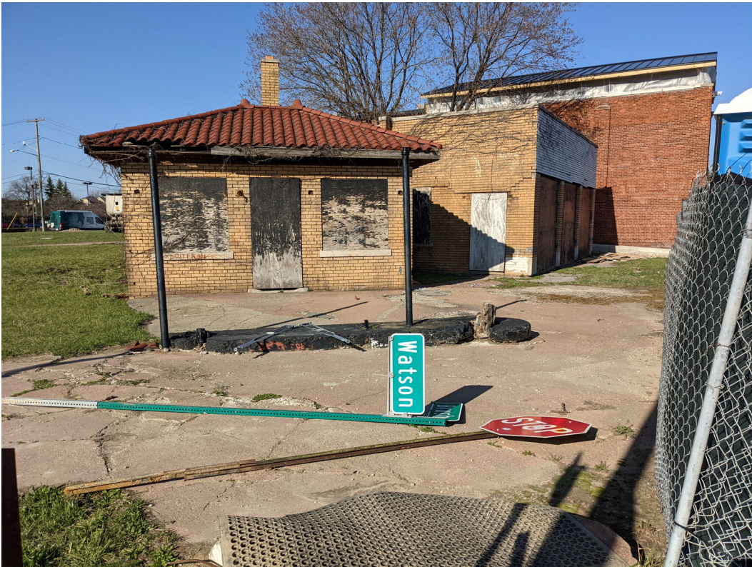
View of filling station at Watson and Brush immediately adjacent to the site. This view is the same orientation as the red arrow on page 2.. Staff photo, March 29, 2021.
