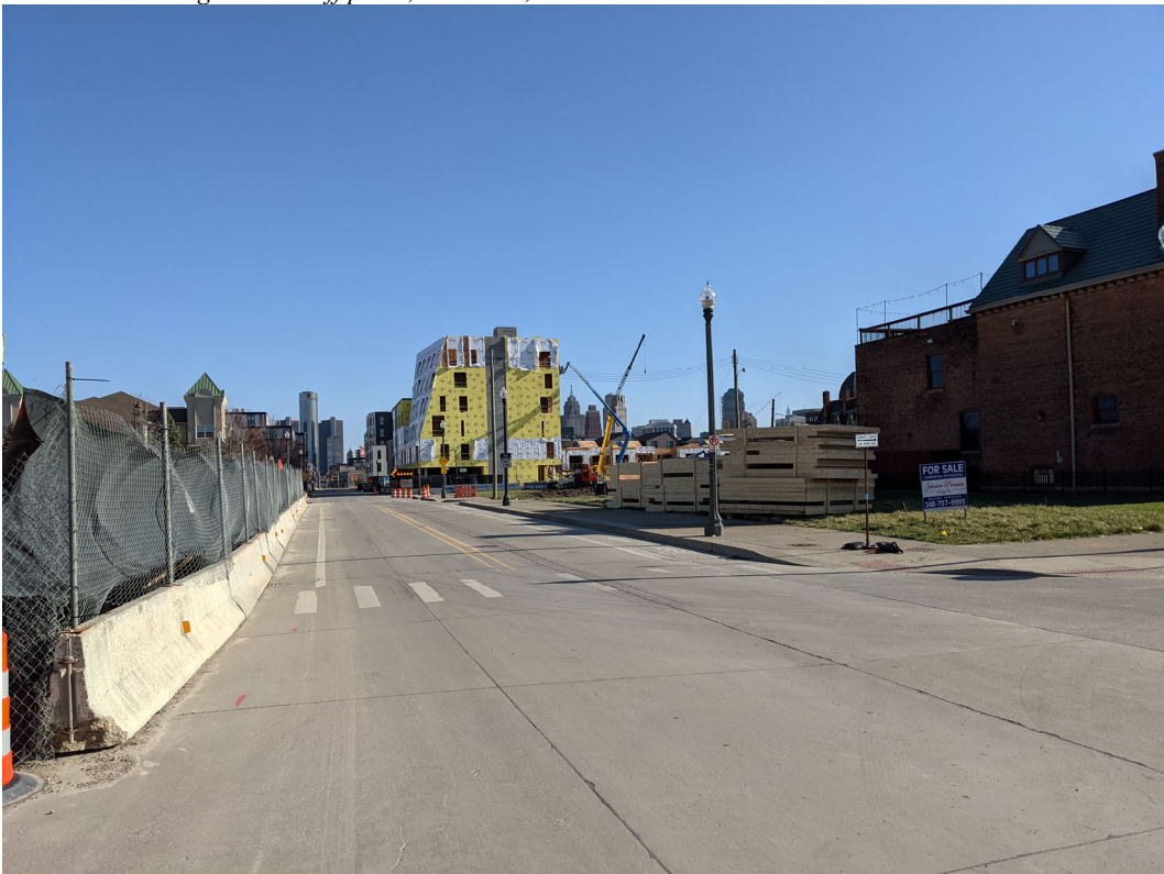
View to south along Brush. Development site visible at left. Staff photo, March 29, 2021.
